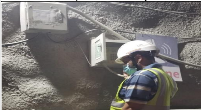
Checking effectiveness of communication Adit#1 by DHC OHS
