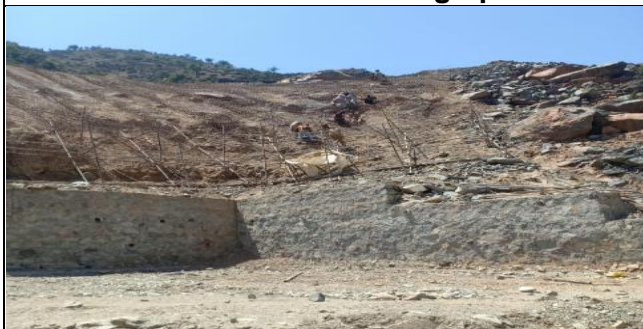
Slope Protection Of Nasirabad Site
