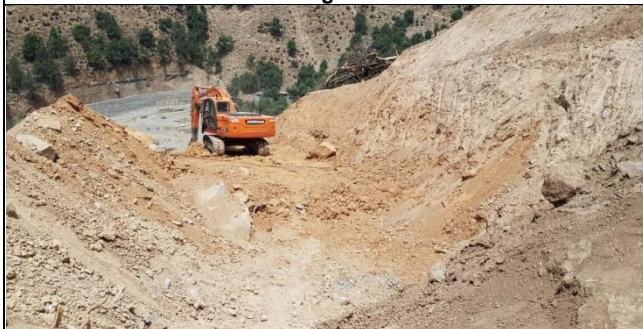
Excavation/Cutting work at Access road to Grid Station.
