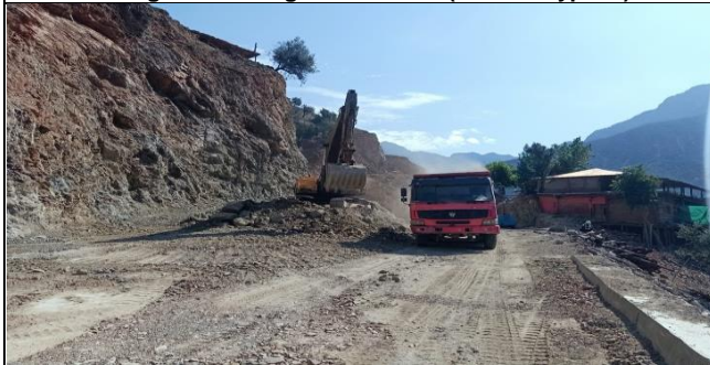
Excavation of Local Access Road K11+600 (RAR-01)
