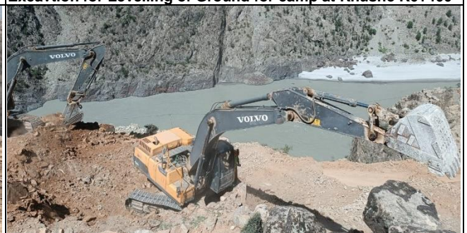
Excavation at K28 access Road
