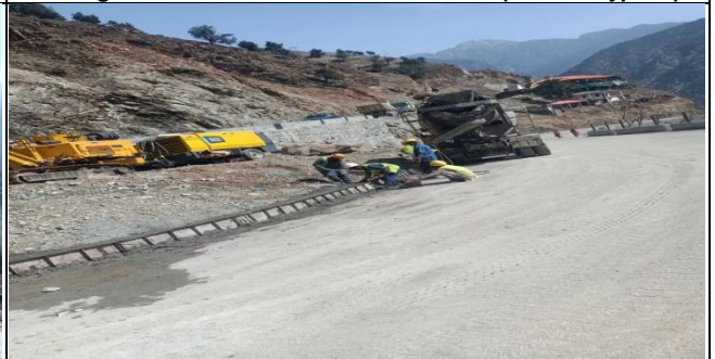
Concrete of Road Side Drain K10+400 (RAR-01)
