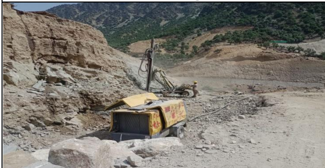
Drilling for Blasting activity at K6+450
