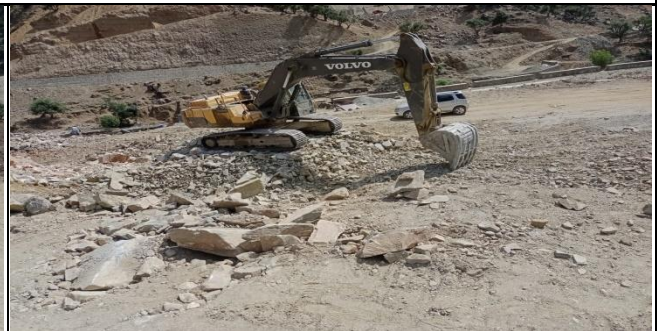
Excavation for Levelling of Ground for camp at Khushe K6+400
