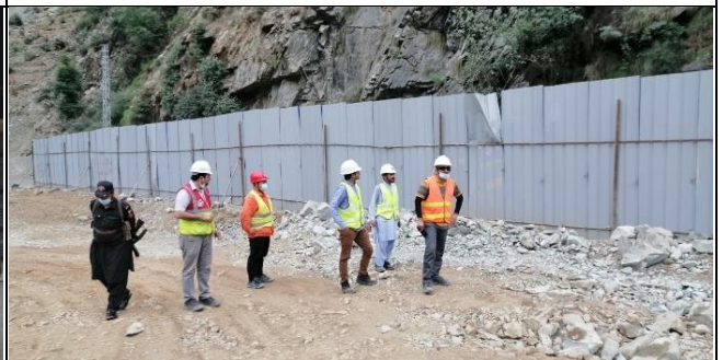
Inspection of KKH boundry fence by DHC OHS at CR9
