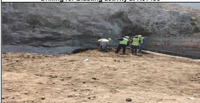
Backfilling above K3 Tunnel Inlet portal
