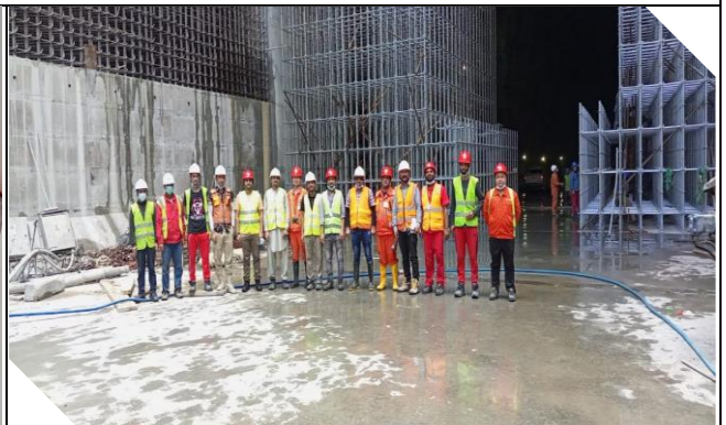
Joint site inspection by DHC OHS at DTA inlet CGGC
