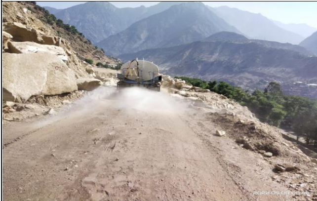
Water Sprinkling at RAR-01, Komila Bypass Contractor Name: CCECC
