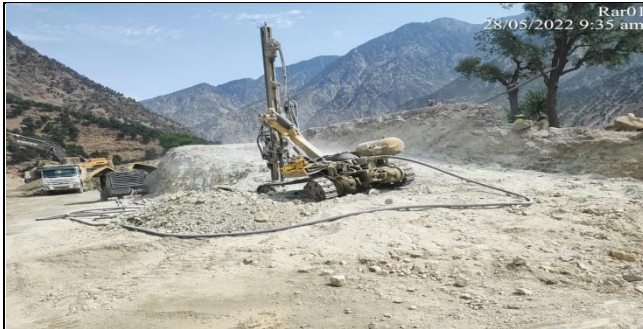
Drilling for Blasting End Section (Komila Bypass)
