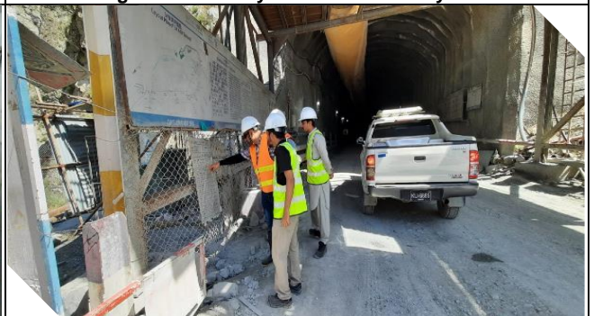
Checking of tunnel air quality at Adit#1 by DHC OHS
