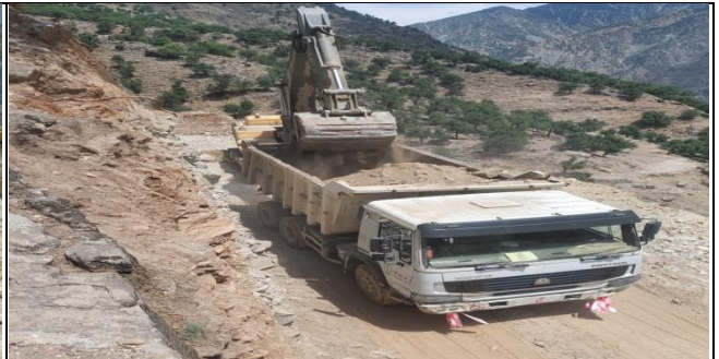
Loading of Excavated Material End Section (Komila Bypass)
