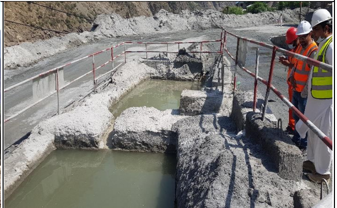
Inspection of Sedimentation Pond at CR-02; Contractor Name: CGGC
