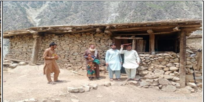
Verification of house for SMR package by FVC in Pani Bah Access Road on 20-5-2022
