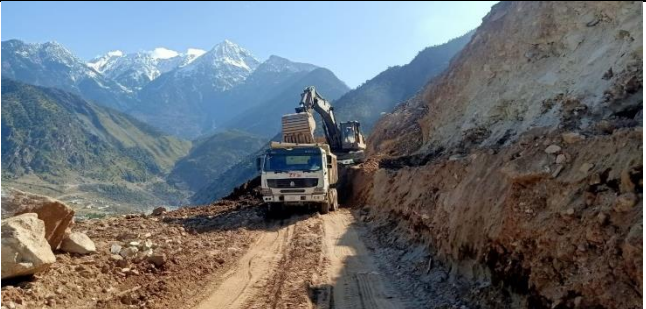
Excavation Catch Point K0+450 Komila Bypass
