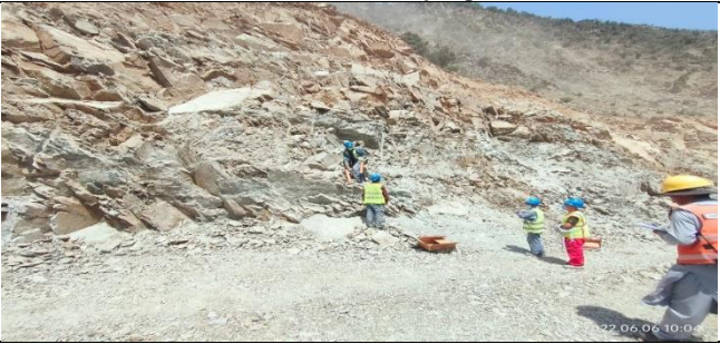
Charging for Blast at K12+990 ~ K13+050
