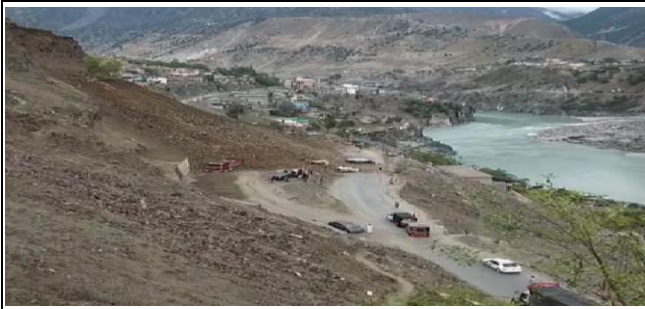
Land Slide Start Section Komila Bypass
