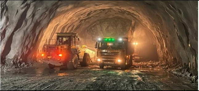
TRT-01 (CT-02) mucking & scaling
