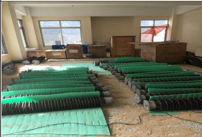
Placement of switch gear equipment in Control House building
