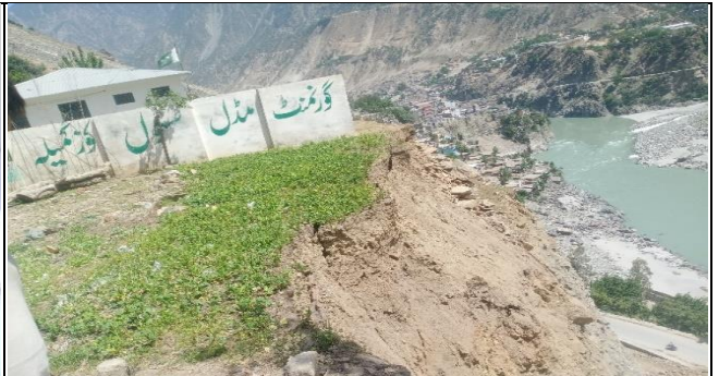
Land sliding and erosion adjacent to GMS Kuz Komila
