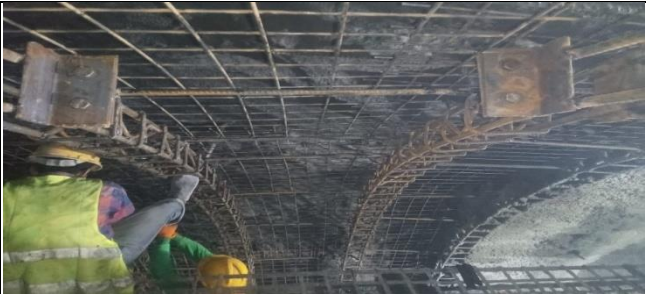
K4 Tunnel nstallation of lattice girders and wiremesh K4+313 to 4+316
