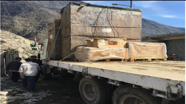
Shifting of Panels from store to Grid Station
