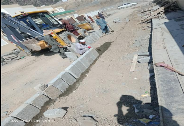
Fixing of curb stone along s1 road
