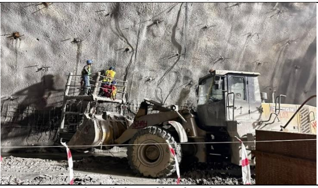
Installations of bearing plates
