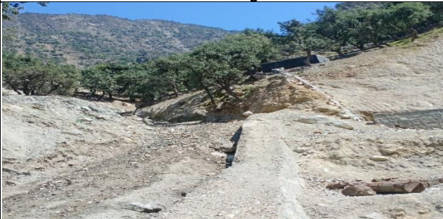
The incompleted Protection wall at Rv Khushi-02 Link-01 (7-4-2023)
