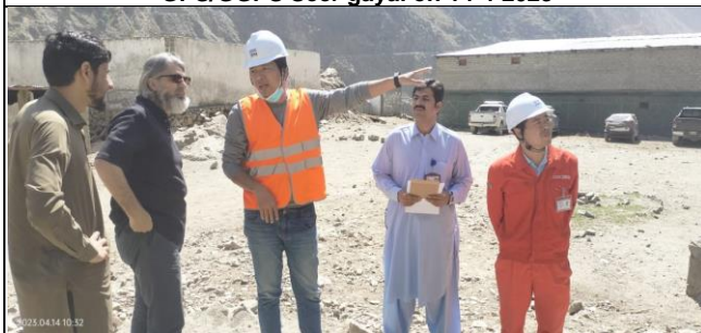
Briefing by the CGGC PM RAR-02 about the layout of access road at Seer gayal on 14-4-2023
