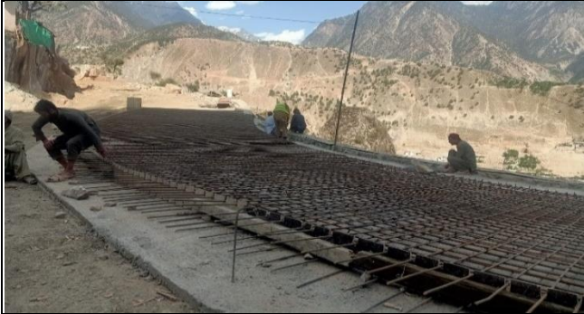
Steel Fixing For Causeway K1+356
