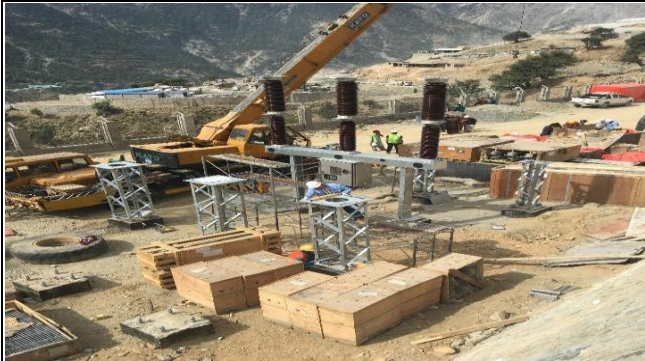
Installation of switch gear equipment on both terraces of Grid Station
