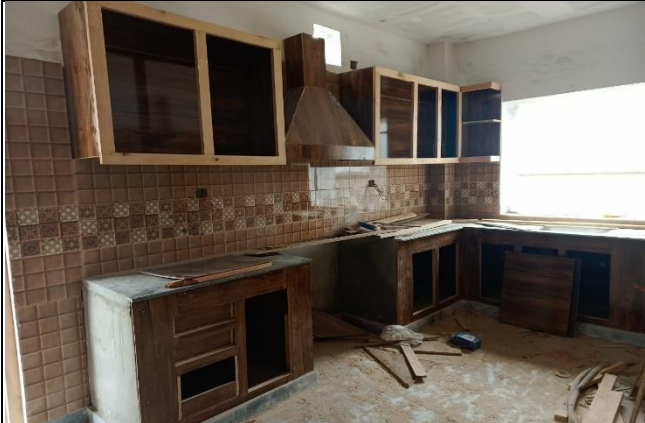
Kitchen cabinet work at cat 2 is in progress
