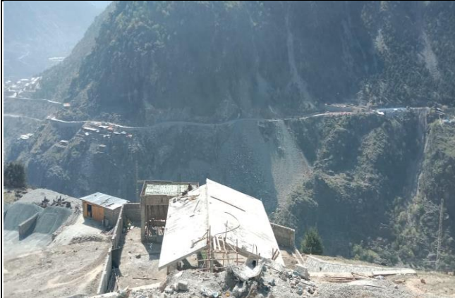
Block masonry at mosque is in progress
