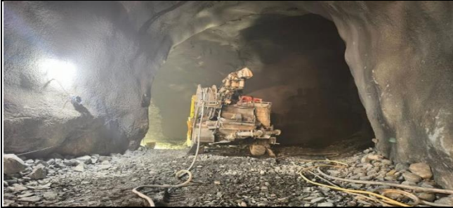
TRT-01 (CT-01) shotcrete
