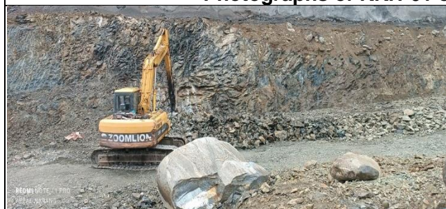
Slope trimming with jack hammer at Zero Point 3rd Bench RD=K1+500-1+550
