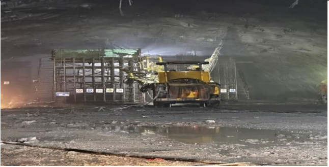
PH Drilling for PS tendons
