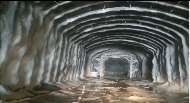
Left Bank Traffic Diversion Tunnel Date 15-04-2023
