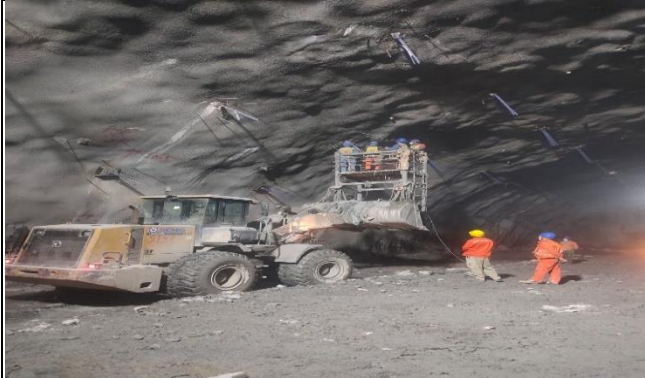
Preparation for installation of Formwork for head block of PS tendon
