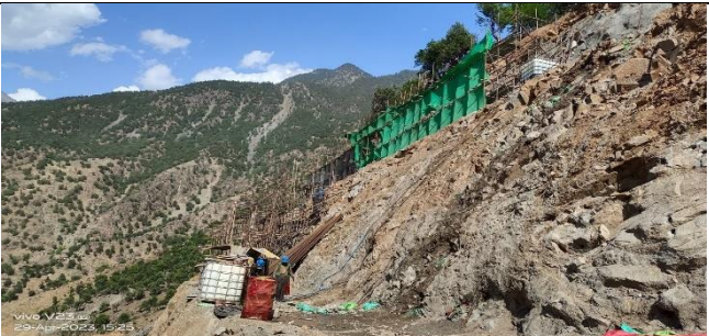
Left Bank Cable Crane Date 29-04-2023
