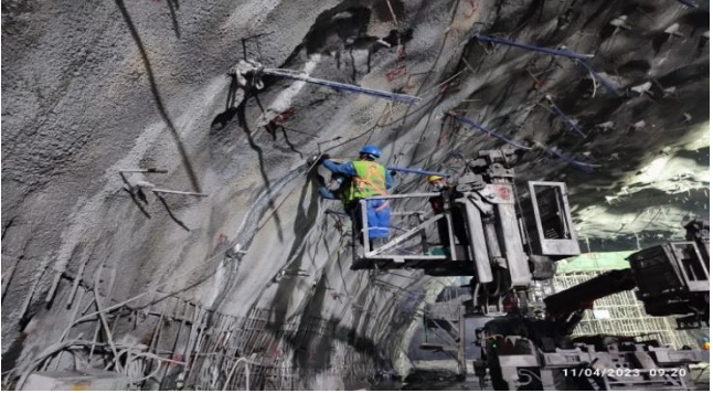
PH. packer grout for ps tendons
