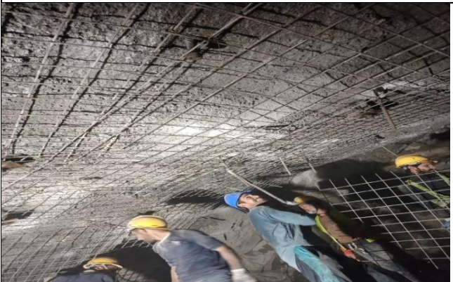
Logro-A tunnel Fixing of wire mesh at K9+463-9+466
