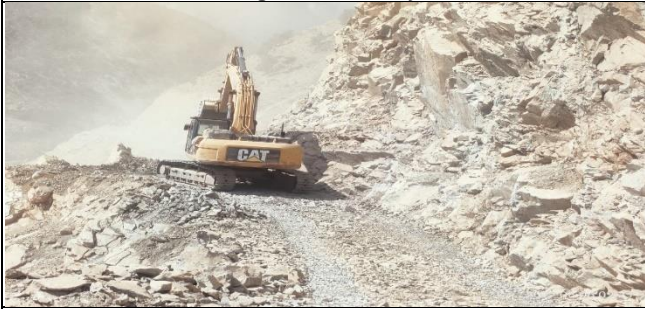
Excavation at K12+960
