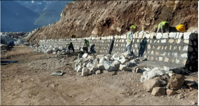
Breast Wall Work in progress
