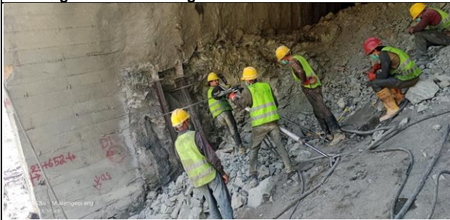
Dugah Tunnel drilling for rock bolts
