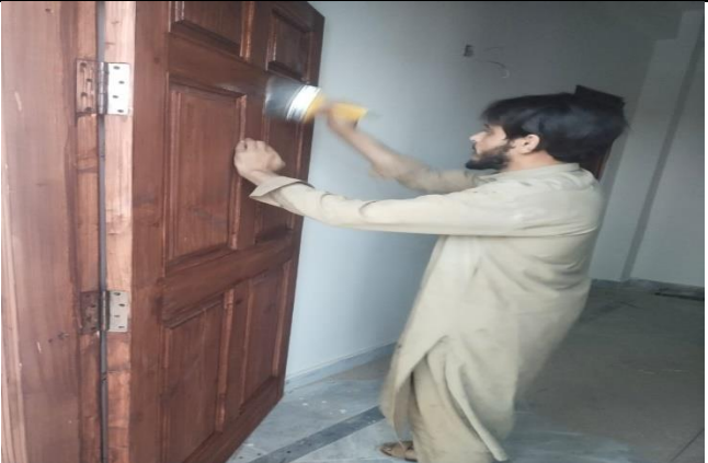
Door poishing work cat 2
