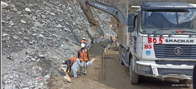
Formwork and laying of RCCP Khuhse Access Road
