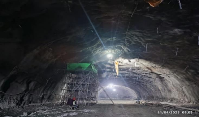
TC drilling for Extensometer
