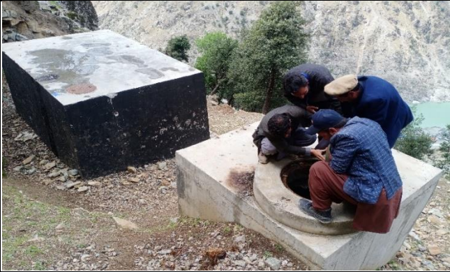
Inspection interior of filter tank at Rv uchar-01
