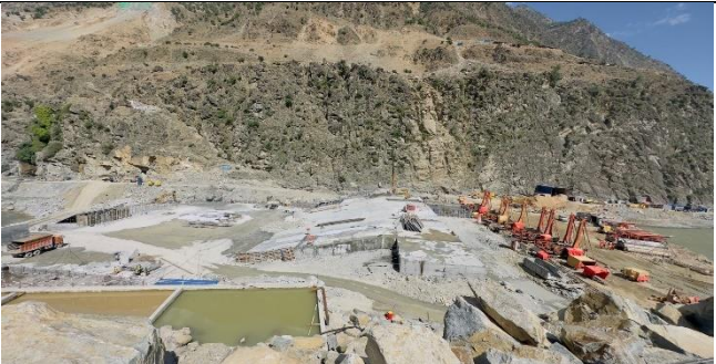
Starter Dam Date 17-04-2023
