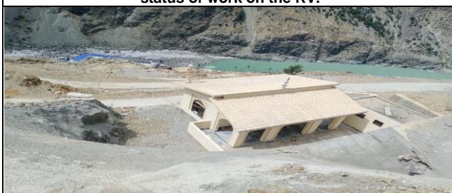
New constructed mosque at Rv nasirabad-01 (5-4-2023)
