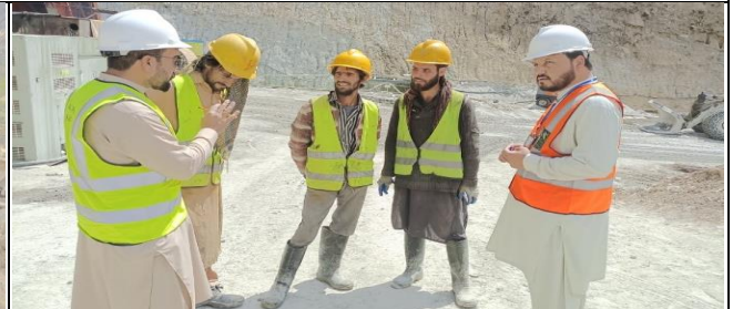
Awareness session with labor at K9 tunnel on 10-04-2023
