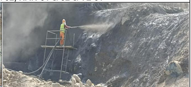
Shotcrete at Zero Point K1+415
