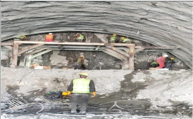
Logro B tunnel K11+894 Charging for blast
