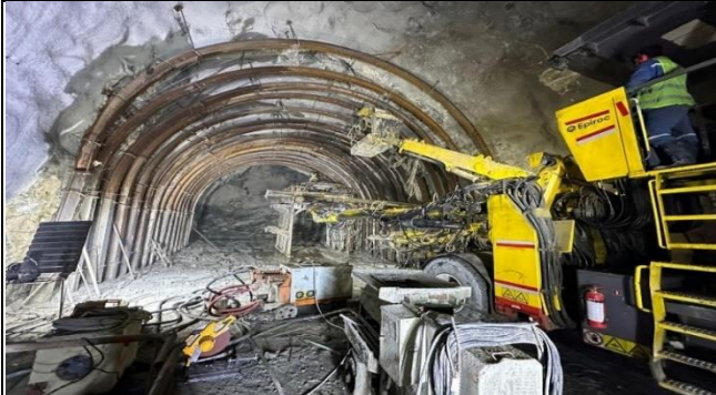
PAT -02 drilling for anchor bars & installation of rebar mesh
