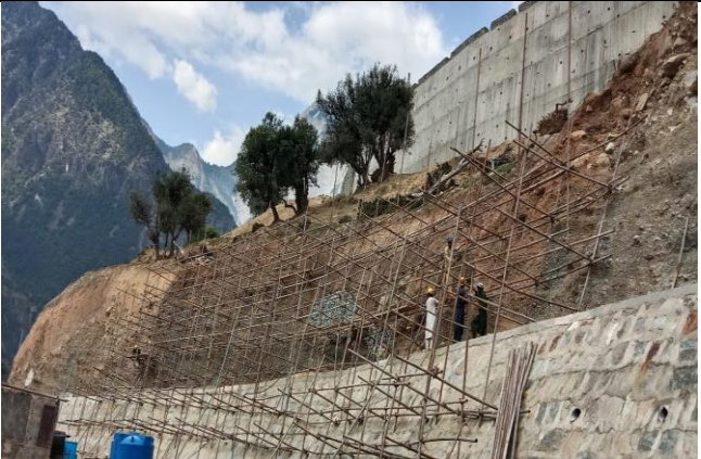
Slope protection work is in progress at Choochang site 1
