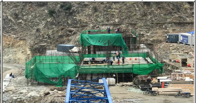
MW-01- Civil work at Uchar Crushing plant aggregate production area
