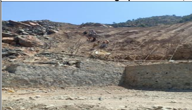
Slope Protection Of Nasirabad Site
