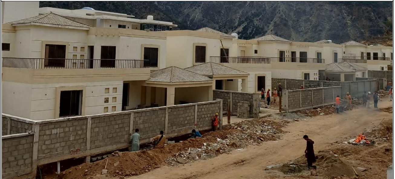
Residence Cat-1 Construction of Boundary Wall in Progress
