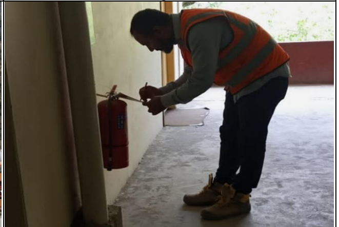
View of monthly fire extinguisher inspection at DHC Office
