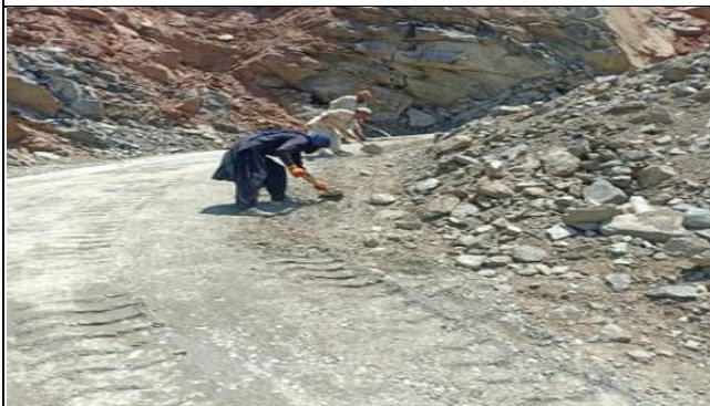
Road Work Nasirabad site 02
