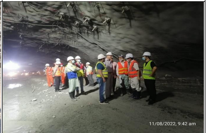
View of DHC, WAPDA and WB higher management visit to MW02
