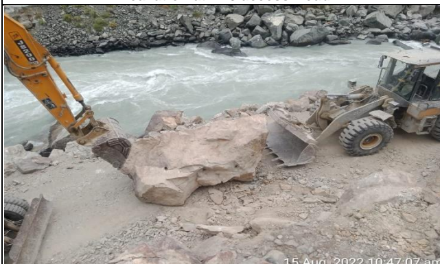
Excavation at Kandia Access Road
