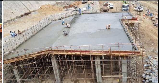
Slab concrete of Control House building
