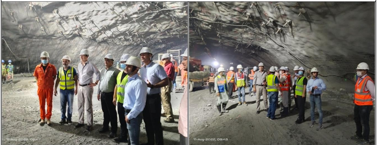
World Bank Team Visit to DHPP Underground Works on 11th of Aug 2022
