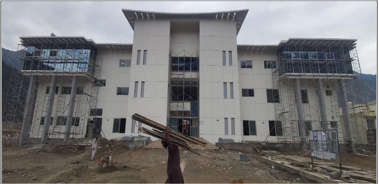
Glass Work and Paint Works in Progress of WAPDA Project Office
