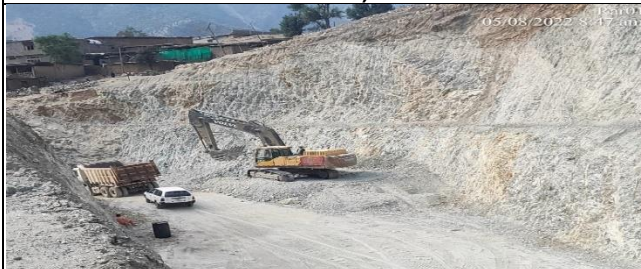
Excavation & Loading K2+180 in progress (Komila Bypass)
