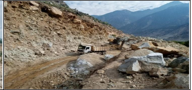
EXCAVATION & LOADING K0+650 (KOMILA BYPASS)
