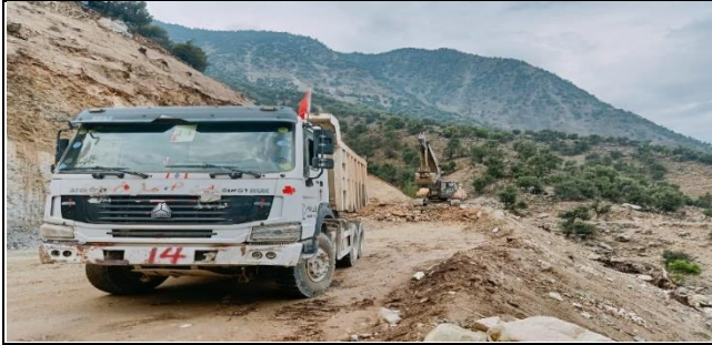
EXCAVATION & LOADING K2+050 in progress (KOMILA BYPASS)
