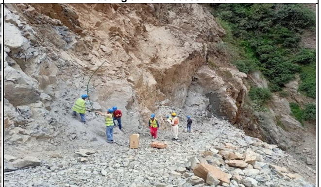
Charging for Blast at K13+250 ~ 290
