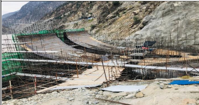
MW01- Formwork of DTB
