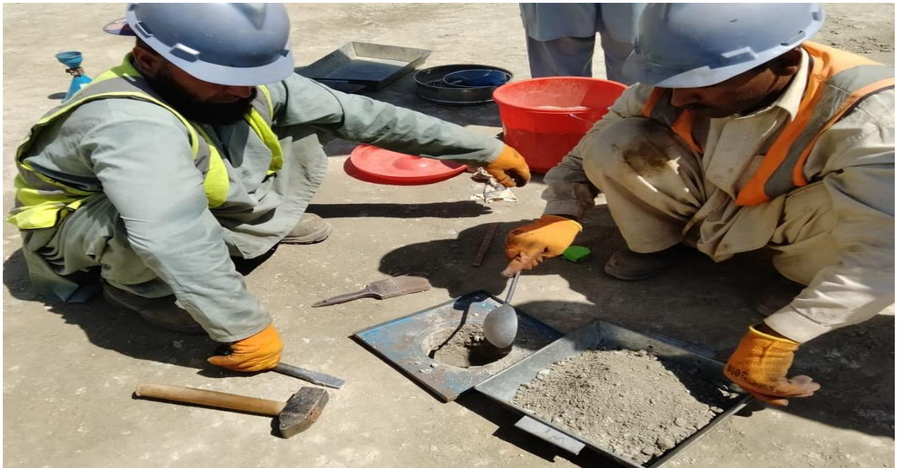
Figure 1 FDT Test for Terrace # 8
