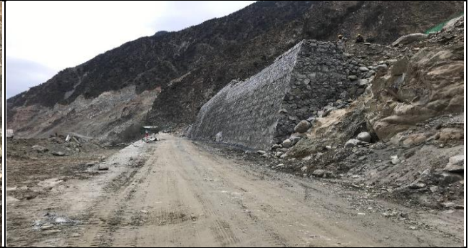
MW01-Retaining wall construction at aggregates staking area of Uchar Crushing Plant (22.08.2022)
