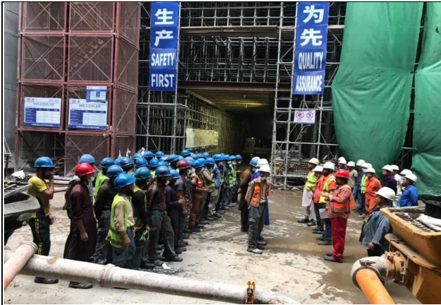
View of routine TBT by CGGC at MW01
