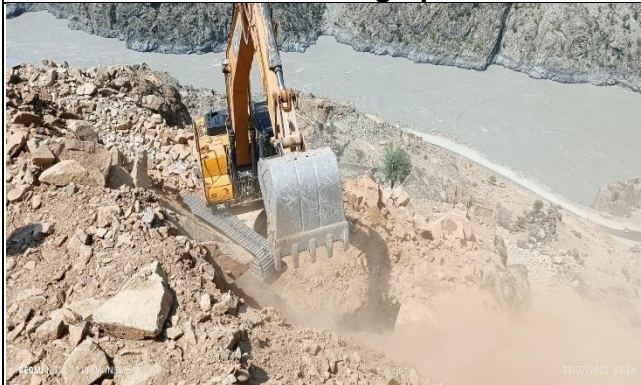
Excavation at K28 access Road
