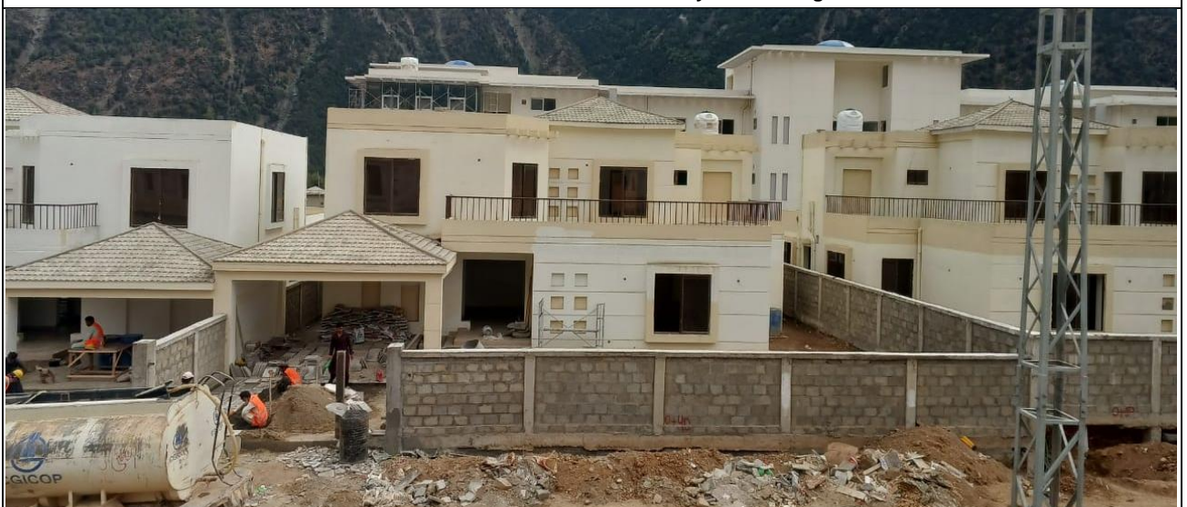
Residence Cat-1 Construction of Boundary Wall in Progress
