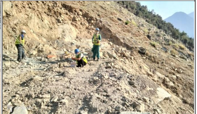
Blasting at K31 Access Road
