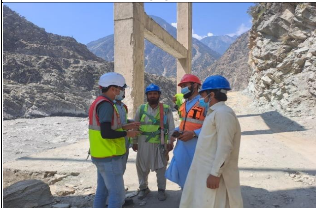
View of routine site walkthrough visit by DHC OHS
