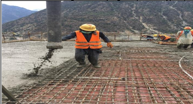
Slab concrete of control house building
