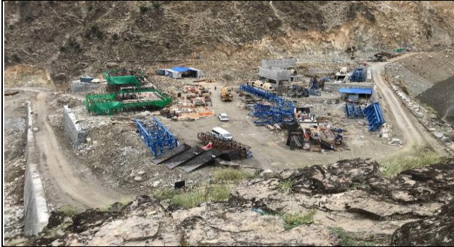
MW01-Fixing Equipmen at Uchar Crushing Plant aggregates production area (22.08.2022) (1)
