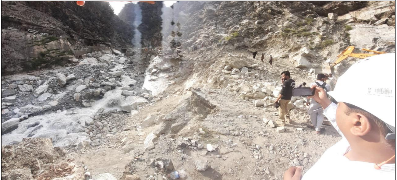
On 30th of Aug 2022 Zaid Khwar Road All Washed away after Flood of 24-27 th of Aug 2022
