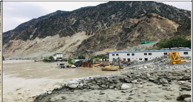
KKH01- CCECC concrete production camp inundated
