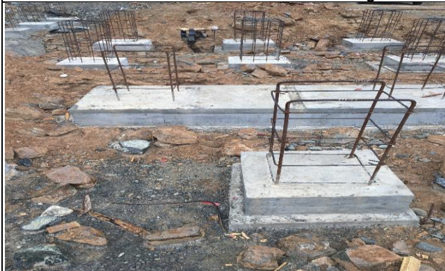
Foundation concrete of switch gear equipments
