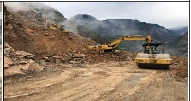
MW02- Excavation for Intake on left bank
