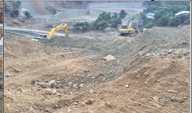
Excavation/Cutting work at Access road to Grid Station.
