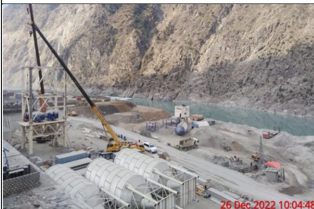
Recovery of machinery and batching Plant from flood material in Uchar
