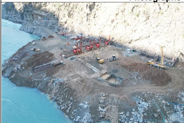
U/S Starter Dam - Right Bank works (MW-01)
