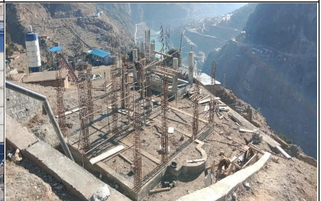
Working of Mosque in progress chochnage site 1
