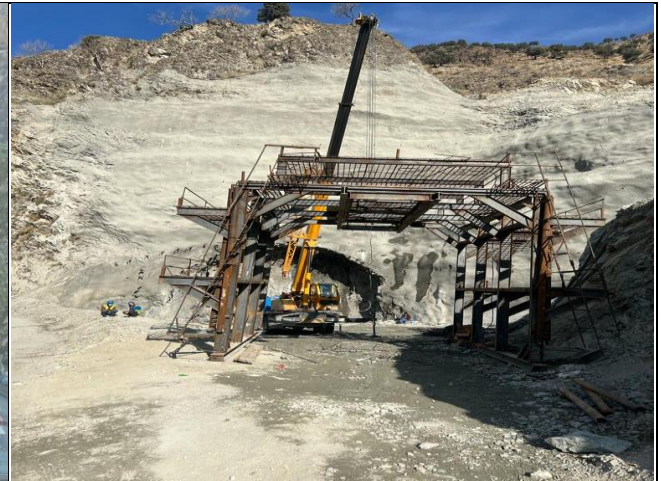
Traffic Diversion Tunnel – Outlet Portal (MW-01)
