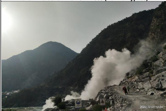
Blasting at Seer Gayal Access Road
