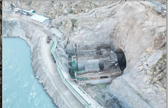
Diversion Tunnel A – Inlet Structure (MW-01)
