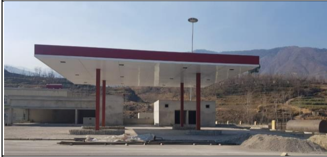
Under construction Fuel station
