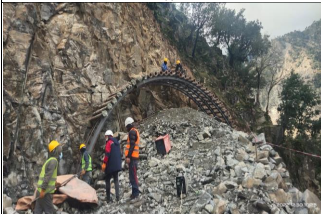
Installation of Serial Arches at Logro-B Outlet
