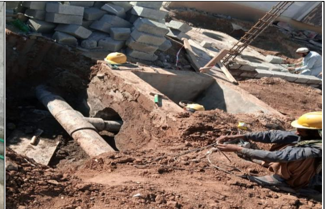
Repair of Main Water Supply at Cat 2
