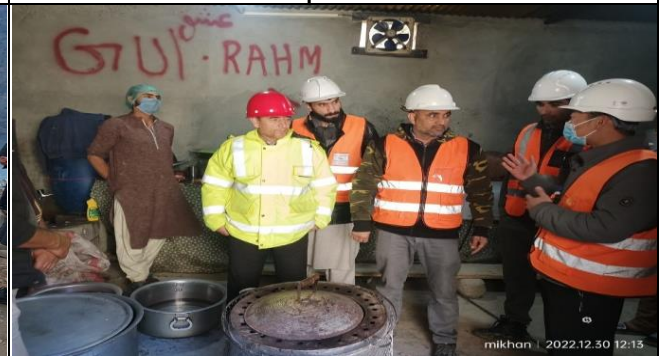
A view of joint inspection with WAPDA and CCECC to KKH01 Camp
