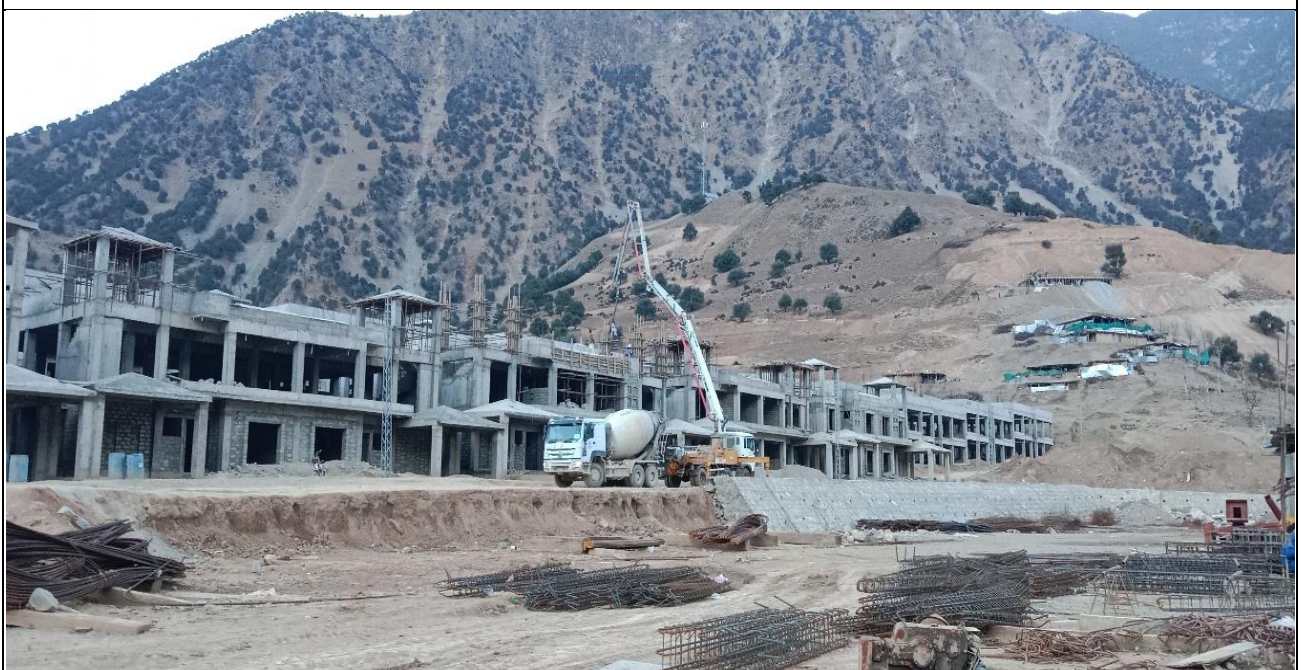
Column concrete of Cat 3
