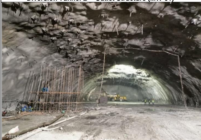
UG Powerhouse Crown Support Work (MW-02)
