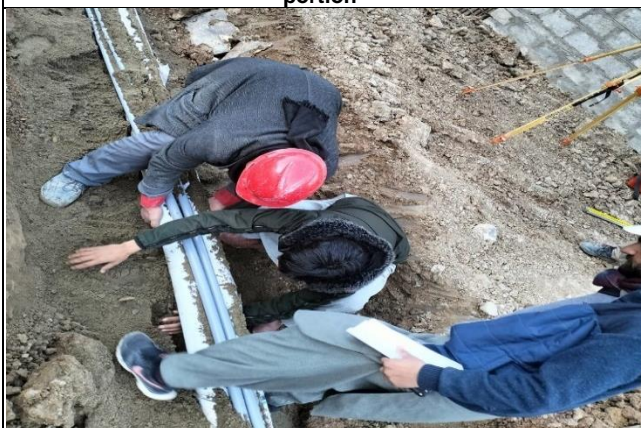
Laying of service cable under ground at cat 2
