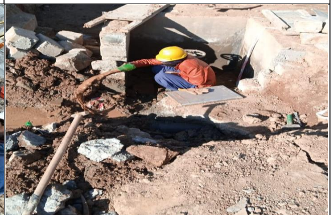
Sluice valve Chamber working at Cat 2
