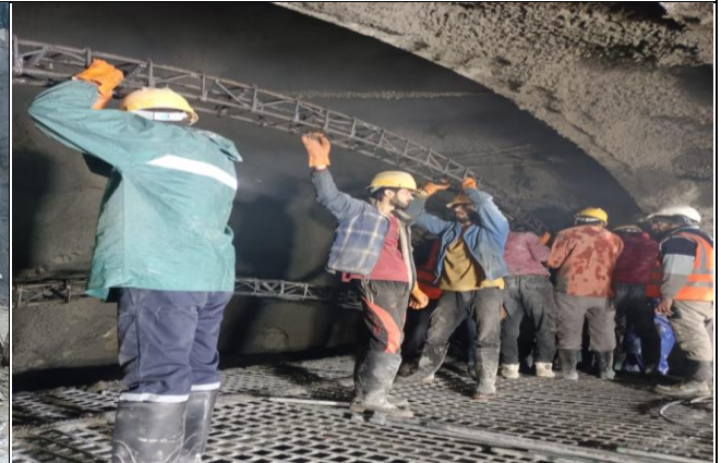
Installation of Steel ribs for primary support in Logro-A RD=K9+245
