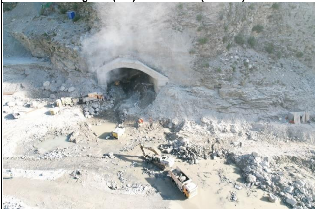
Diversion Tunnel B – Outlet Structure (MW-01)
