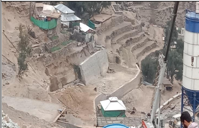
Retaining wall work in progress at kuz chochnage lower portion
