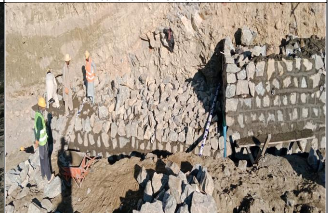
Construction of Breast wall at access road of Grid Station
