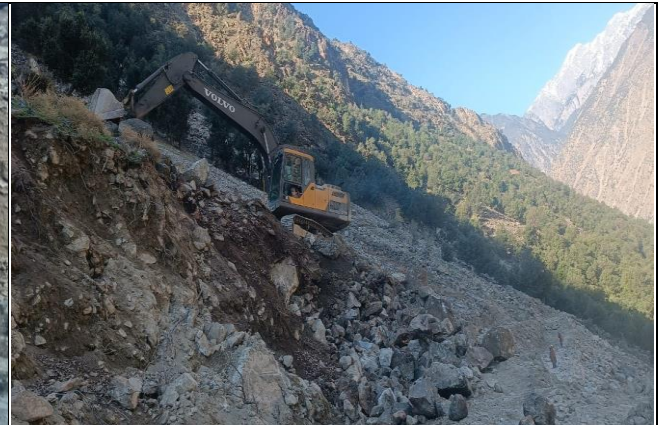
Excavation at K33+800 RAR02
