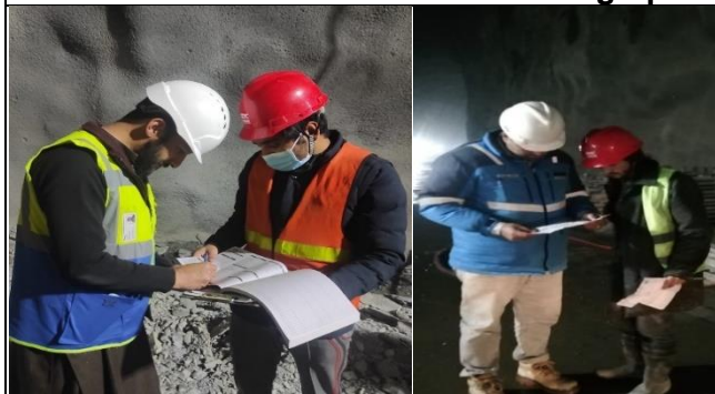
DHC OHS Professionals verifying pre-start hazard assessments at MW01 and MW02
