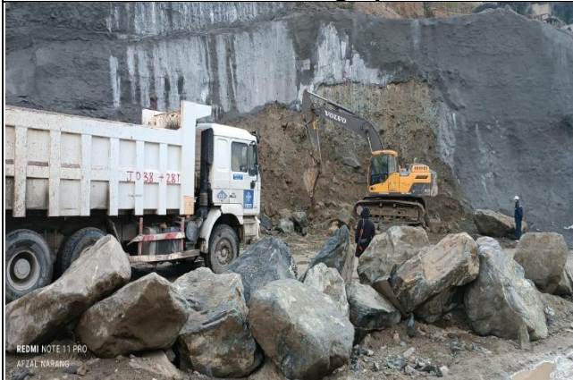
Excavation and loading at Zero Point 3rd Bench RD=K1+450-1+480
