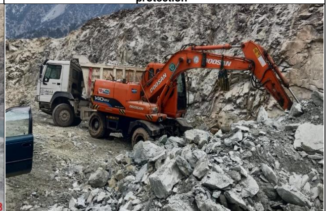
Excavation & Loading of Material K2+190 (KOMILA BYPASS)
