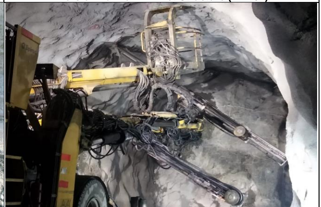
Adit 3-2 Tunnel (MW-01)
