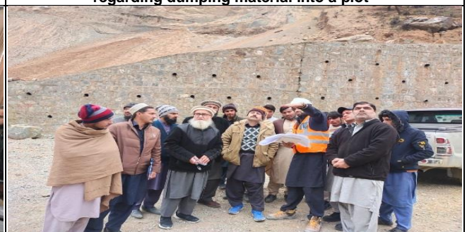
A joint visit with Director (S&R) WAPDA, Chairman IGRC and Infrastructure Team from DHC was conducted to Kuz Chuchang regarding the re-alignment of Access Road for Upper portion.
