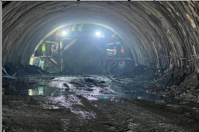
Logro A (K-9) Tunnel inlet (KKH-01)
