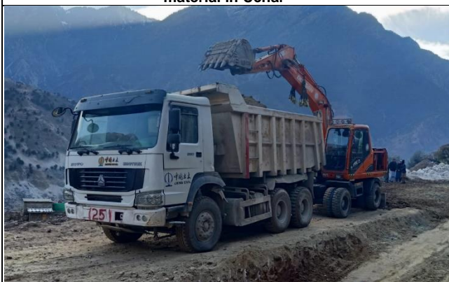
Excavation work for road K1+750 (KOMILA BYPASS)
