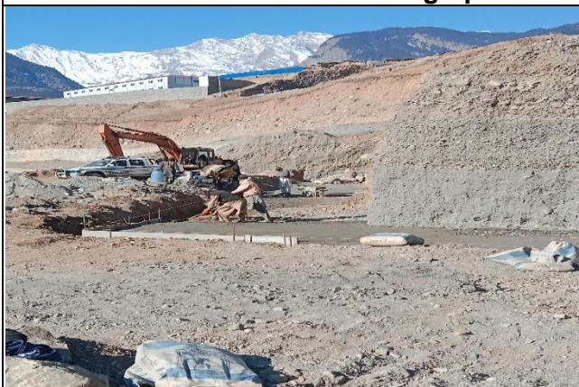
Pouring of concrete Breast wall at chochnage site 01
