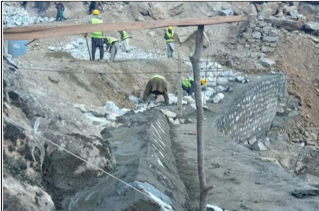
Nullah Protection Works K1+350 (Komila Bypass)
