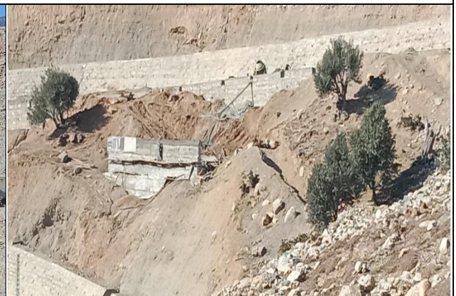
RCC wall in progress chochnage site 01
