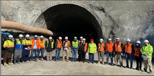
A view of World Bank visit to the CT02 Tunnel – MW02
