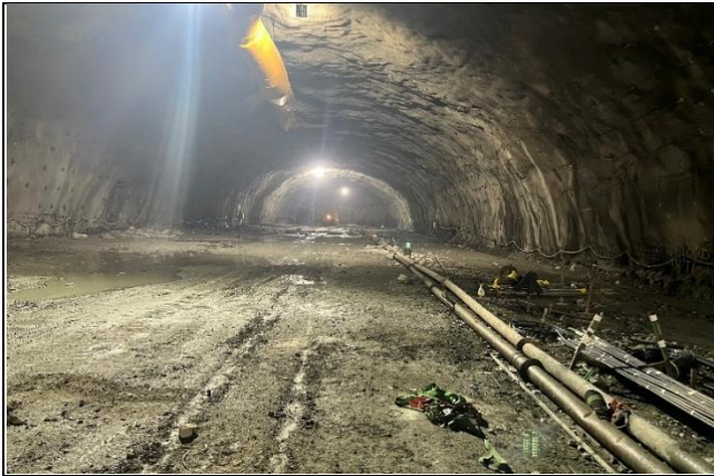
Transformer Cavern Crown Support Work (MW-02)
