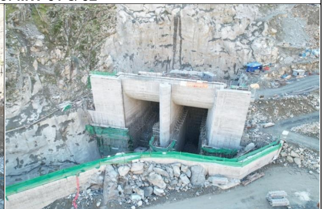
Diversion Tunnel B - Inlet Structure (MW-01)
