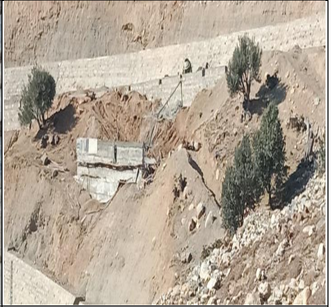
RCC wall in progress chochnage site 01
