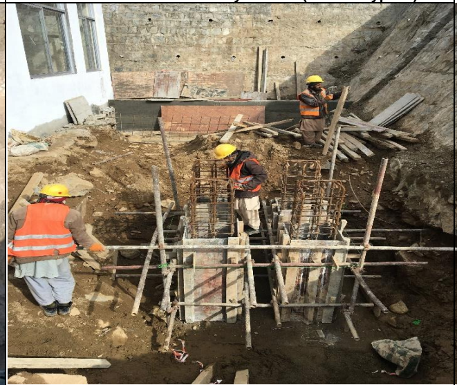
Steel fixing for foundation of Earth Mast
