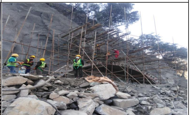
Drilling for rock bolts at Logro-B Outlet
