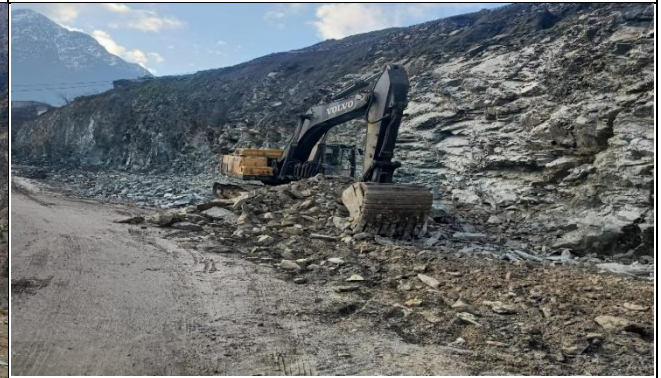
Excavation & Loading of material K2+252 (KOMILA BYPASS)
