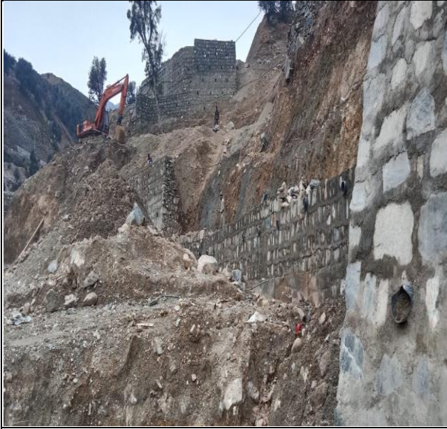
Stone masonry retaining wall is in progress
