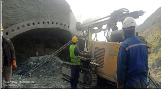
Drilling for advance support Canopy Pipes) Dugah Tunnel outlet.
