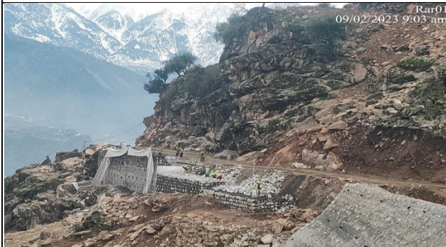
Stone Masonry R/Wall in progress K1+252 (KOMILA BYPASS)
