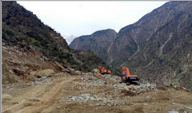
Excavation at K44
