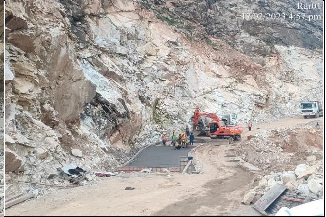
Lean Concrete for causeway K0+900 (Komila Bypass)
