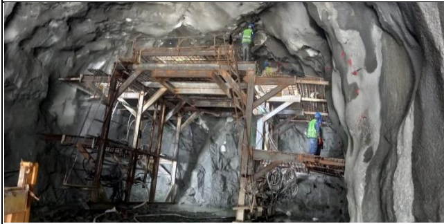
Right bank Diversion tunnel outlet
