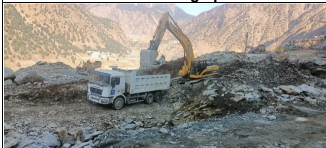
Excavtion and loading at Zero Point 3rd Bench RD=K1+500-1+550
