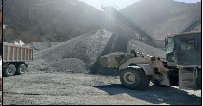
Uchaar Crushing plant
