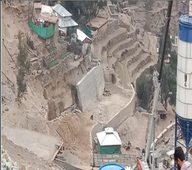
Retaining wall work in progress at kuz chochnage lower portion
