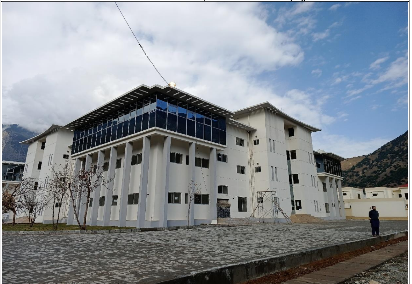
Tuff tile Working Finish in Front of Project Office
