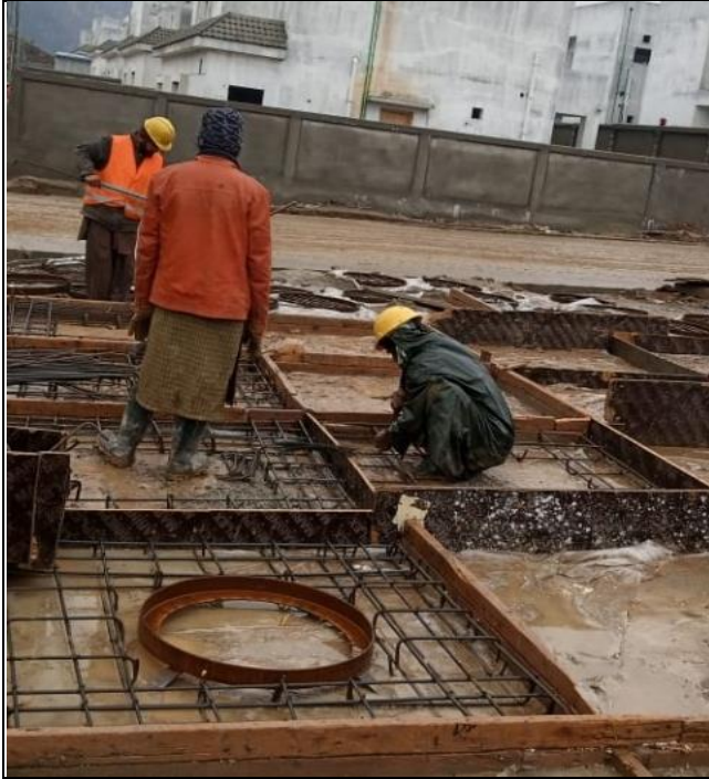
Reinforcement of sluice valve chamber top slab
