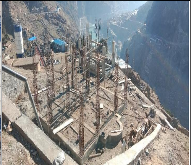
Working of Mosque in progress chochnage site 1
