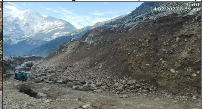
Excavation for slope cutting K0+600 inprogress (Komila Bypass)
