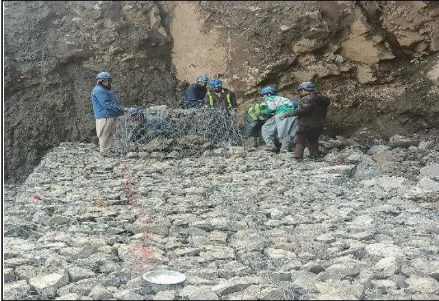
Gabion wall Construction at Siglo K13
