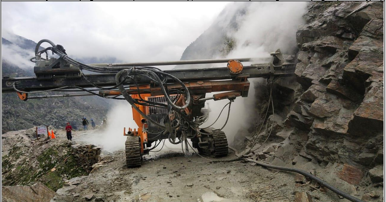
Drilling at Seer Gayal Access Road
