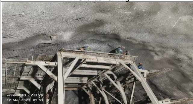
CT2 TRT US wire mesh fixing
