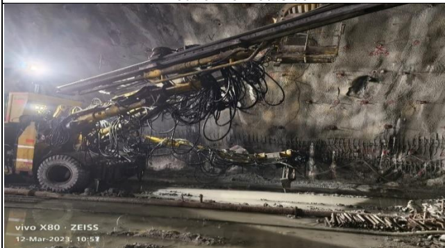
PH PS tendon drilling
