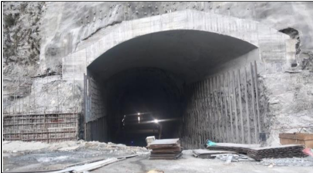
DT-A outlet from outside
