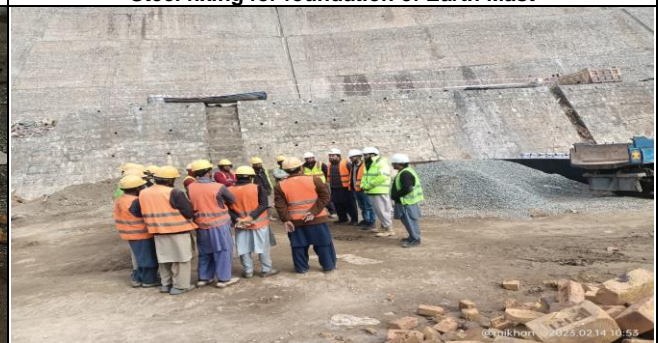
Discussion on safety implementation and improvement at Grid Station site
