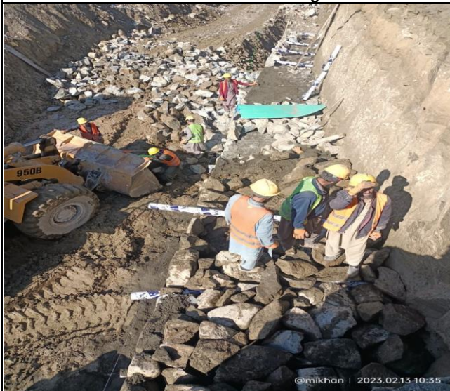
Construction of Breast wall at access road of Grid Station.
