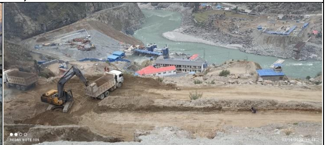
Excavtion work for improvement of Khuhse Bypass road
