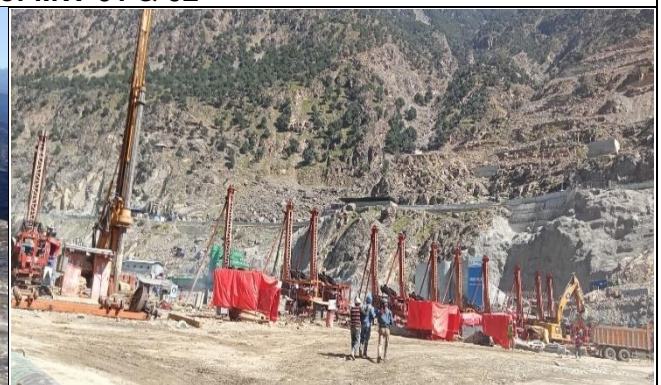
cut off wall
