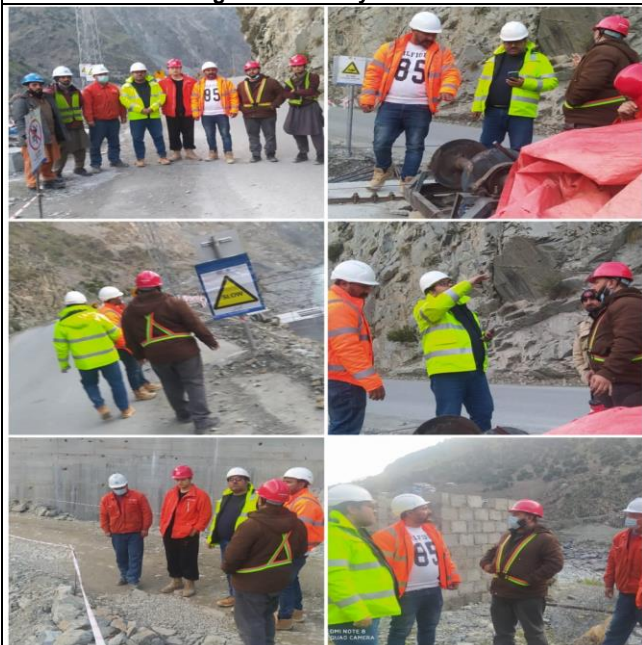
A view of joint inspection conducted by DHC and The Contractor at RAR02
