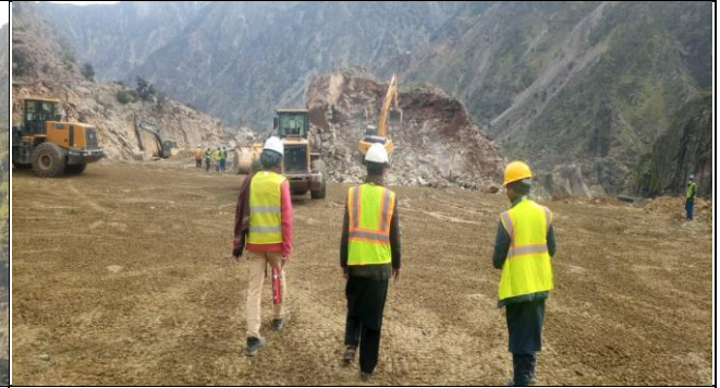
Excavation at Looter Camp
