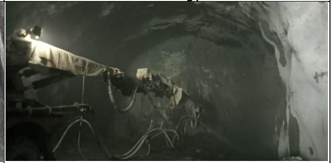
Right bank Diversion tunnel inlet
