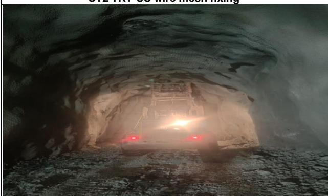
Tailrace 01 Fixing of wire mesh (crown portion)
