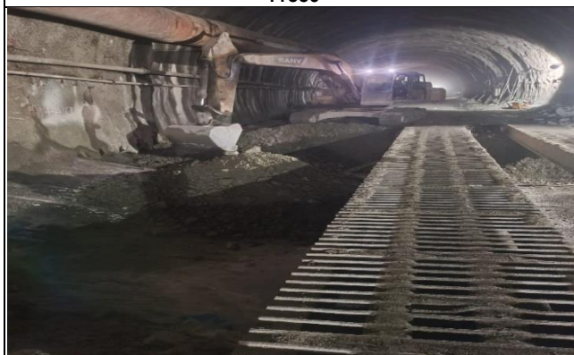
Excavtion for invert arch of Logro-A RD=K9+210-9+216
