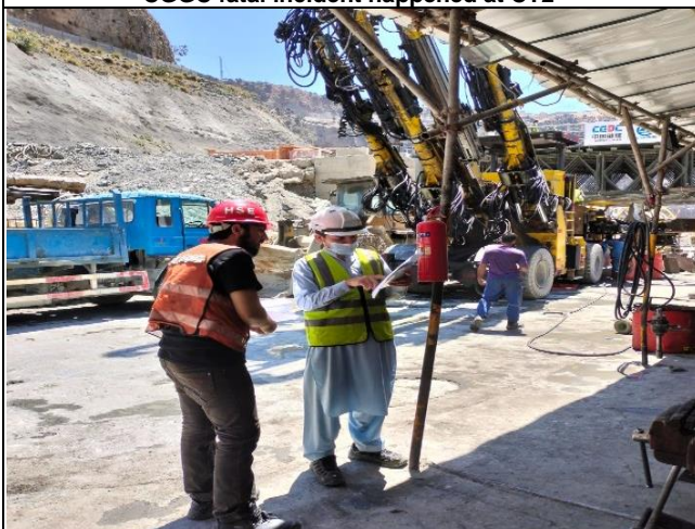
Monthly fire extinguisher inspection of CGGC conducted by DHC OHS at CR9 workshop
