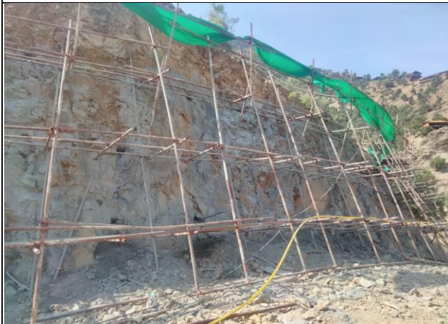
MW-01_Right Bank Excavation for Cable Crane
