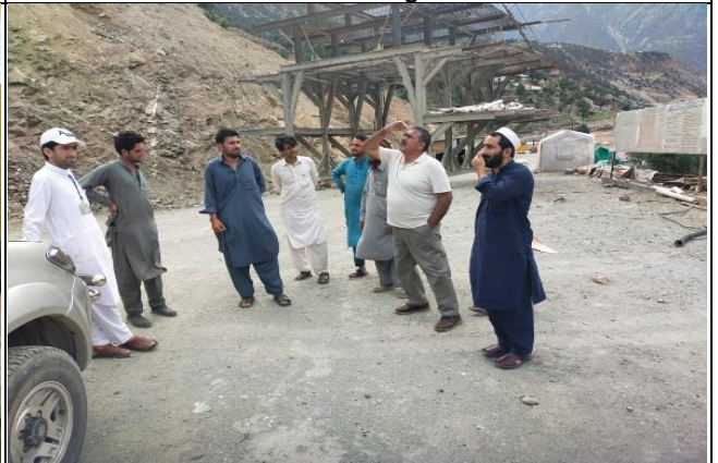
Inspection visits with Advisor R&R WAPDA for Damaged Houses due to Blasting at Tailrace Area
