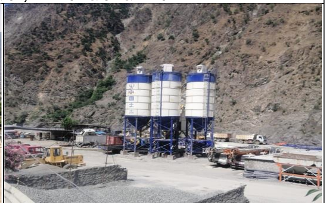
KKH-01_Preparatory Works for Tunnels & Bridges
