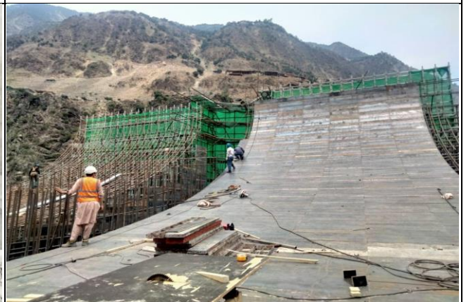
MW-01_Diversion Tunnel-B Inlet slab part
