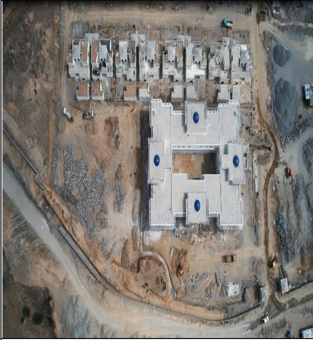
PCI-01R_Finishing work at Project Office and Cat-1 Residences
