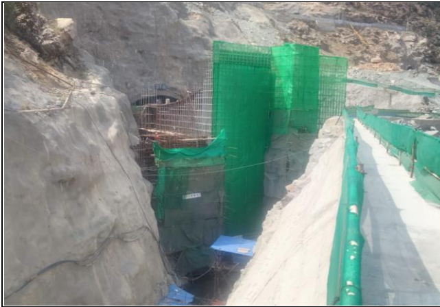
MW-01_Diversion Tunnel-B outside
