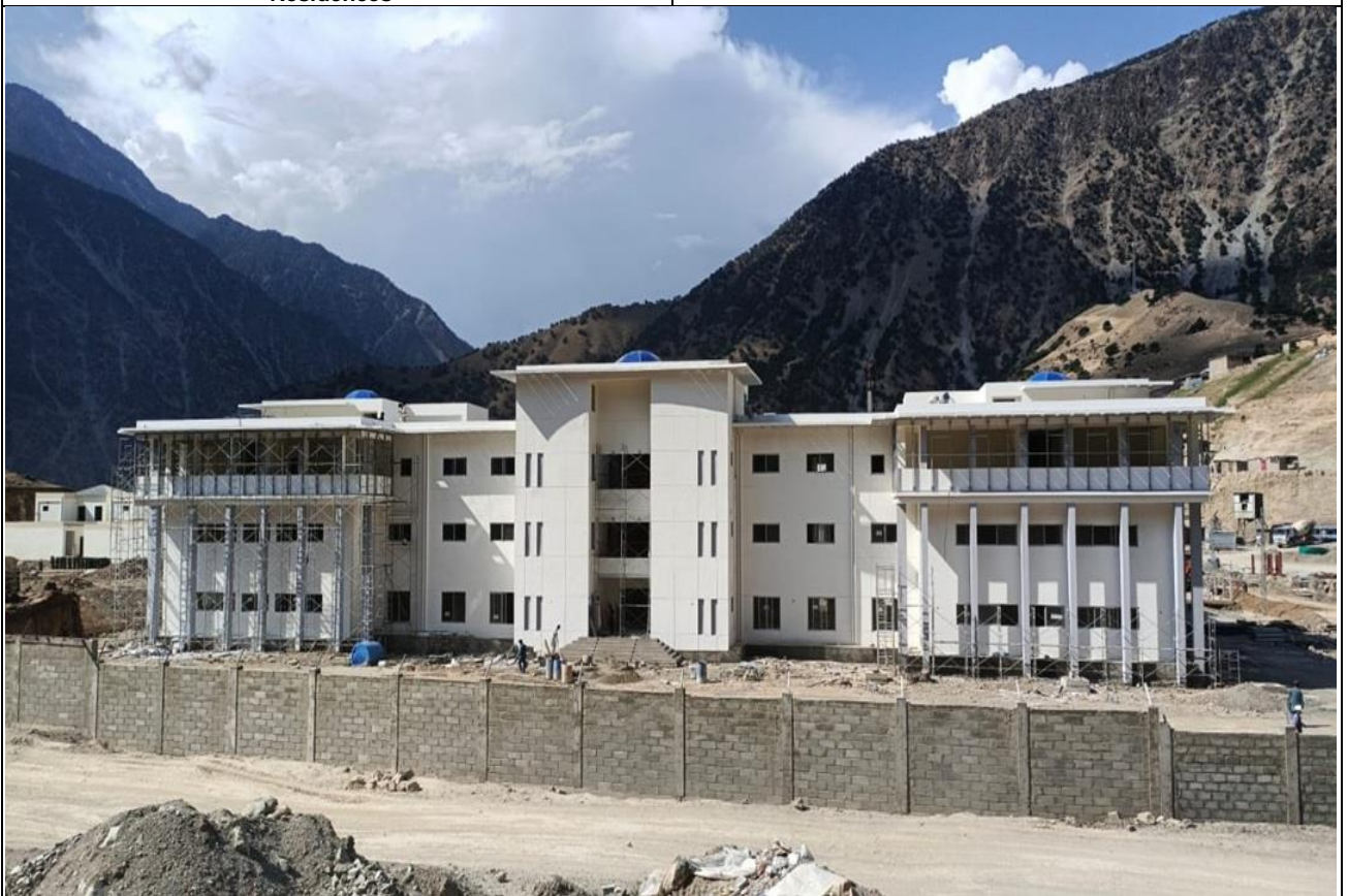
PCI-01R_Finishing work at Project Office Building1
