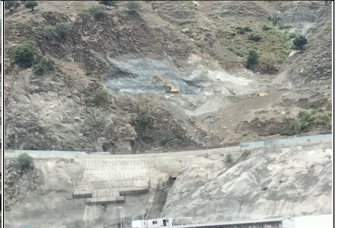
MW-01_ Excavation at Left Bank Traffic Diversion Tunnel Outlet portal
