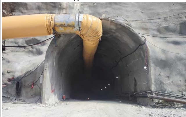
MW-02_Excavation at CT-02 at K0+000
