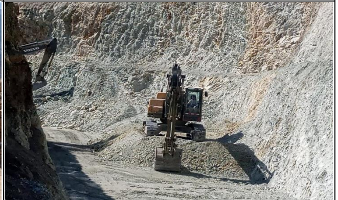
RAR-01 Excavation and loading 2+130
