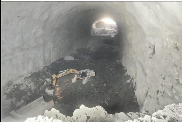
MW-01_Diversion Tunnel-B Down Stream
