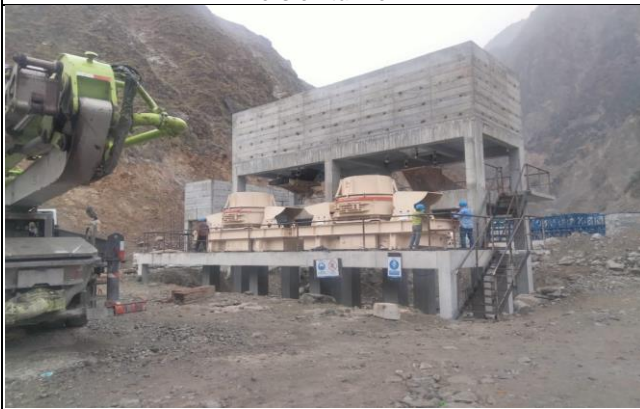
MW-01_Civil work at Uchar Crsushing Plant
