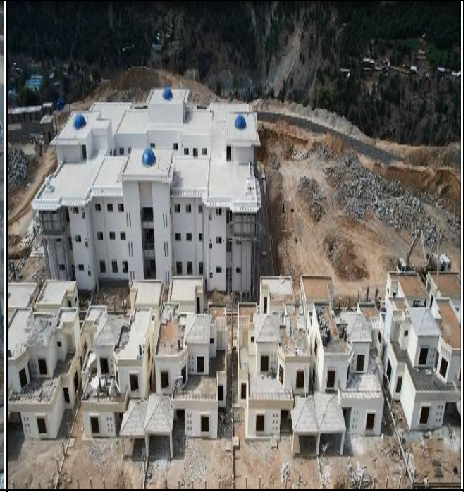
PCI-01R_Finishing work at Project Office Building
