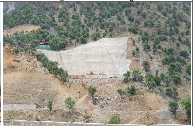
TL-01 Access Road to Grid Station & Control building
