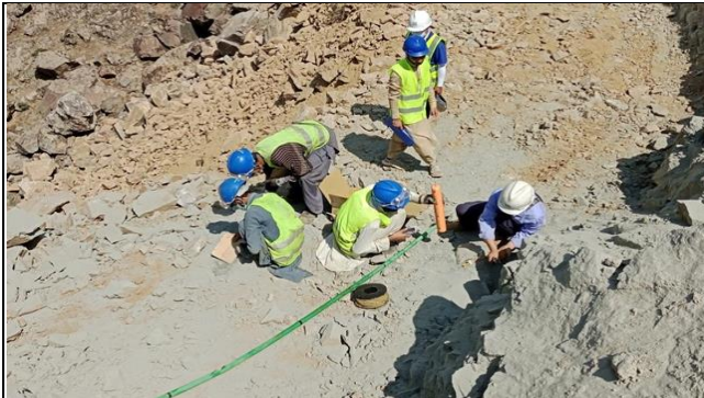
KKH-02 Charging for Blasting at K31 Access Road
