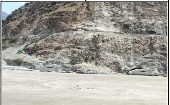
MW-01_Diversion tunnel Outlets from RAR
