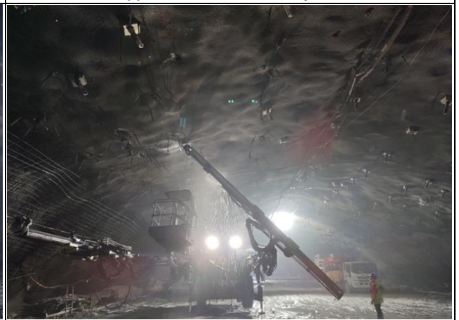
MW-02_Additional Support Work at Powerhouse
