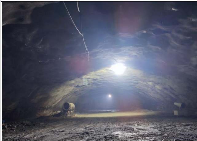
MW-02_Additional Support work at Transformer cavern
