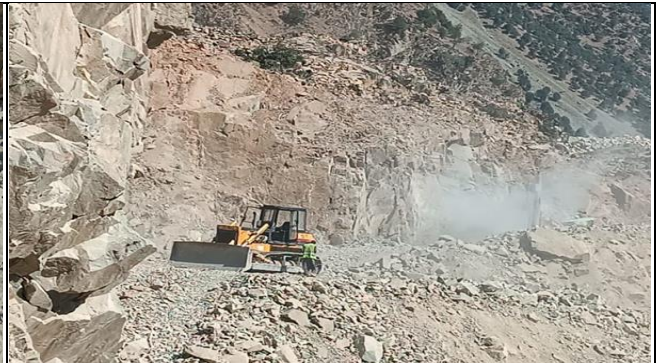
KKH-02 Excavation at K28 access Road
