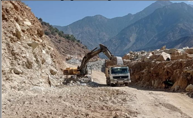
RAR-01 Excavation and loading 0+650
