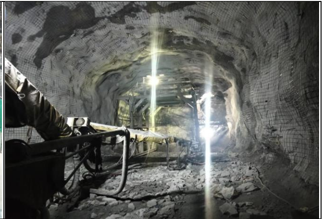
MW-01_Excavation of Left bank Traffic Diversion Tunnel
