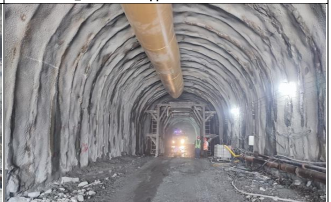
MW-02_Excavation at CT-02 at K0+90m
