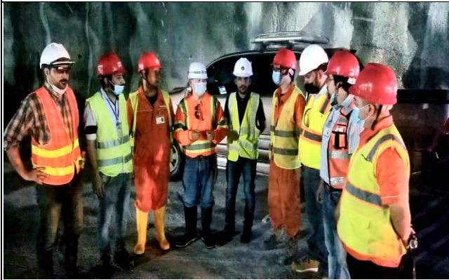
A view of weekly joint site inspection by DHC OHS at DTB
