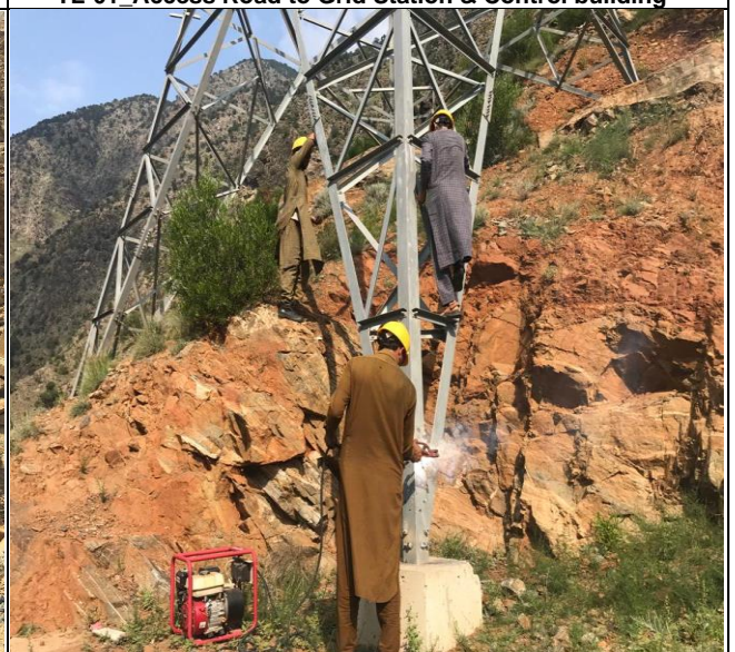
TL-01: Arc welding of nuts and bolts at T-68A
