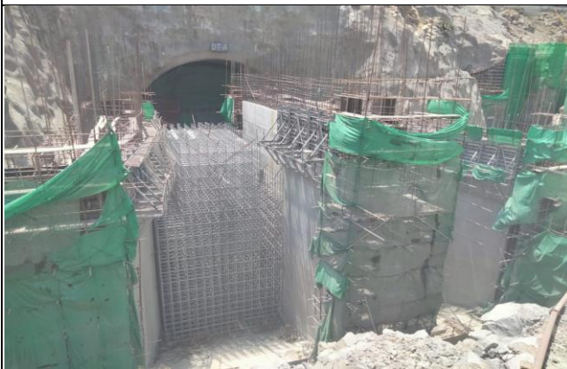
MW-01_Diversion Tunnel-A Inlet outside
