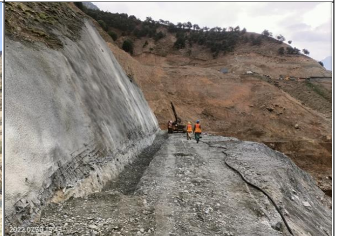
MW-02_Support work for the switchyard at El. 970
