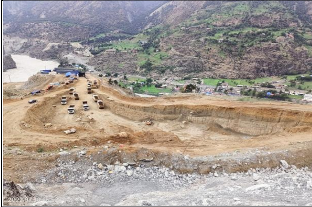
MW-02_Excavation at Switchyard
