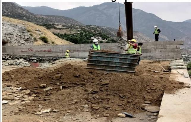
KKH-01_Backfilling Work at K3 Tunnel
