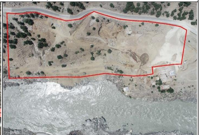
EM-01_Construction of Kass Camp
