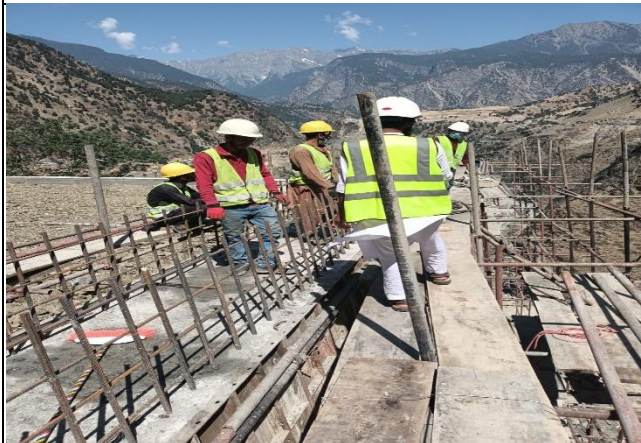
Formwork of Sismic reinforcement wall at K3 Tunnel loutet portal
