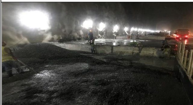
Invert Slab Concrete
