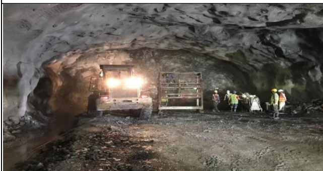
Adit Tunnel at Tailrace
