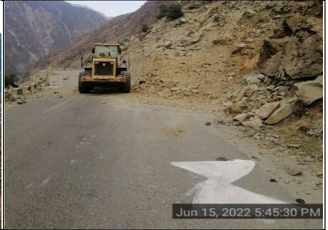
Excavation at K37 Access Road KKH02
