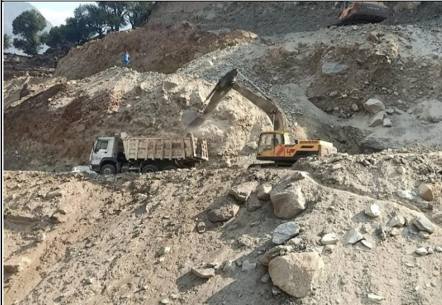
Excavation & Loading around K2(Komila Bypass)
