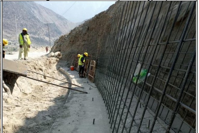
Rebars for B/Wall (Komila Bypass- start section)
