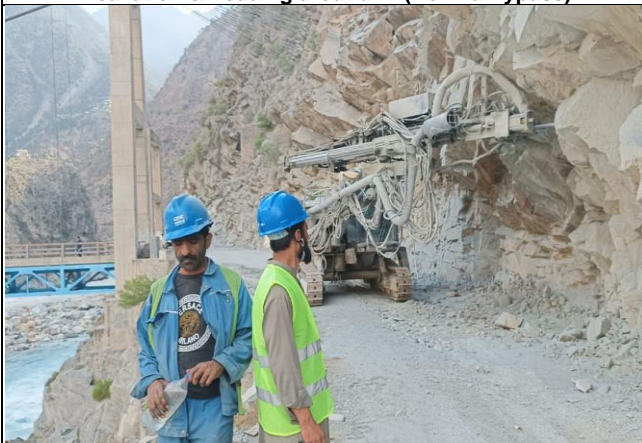
Drilling for Blast at Kandia Bridge Access Road Widening
