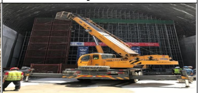
Diversion Tunnel-A inside
