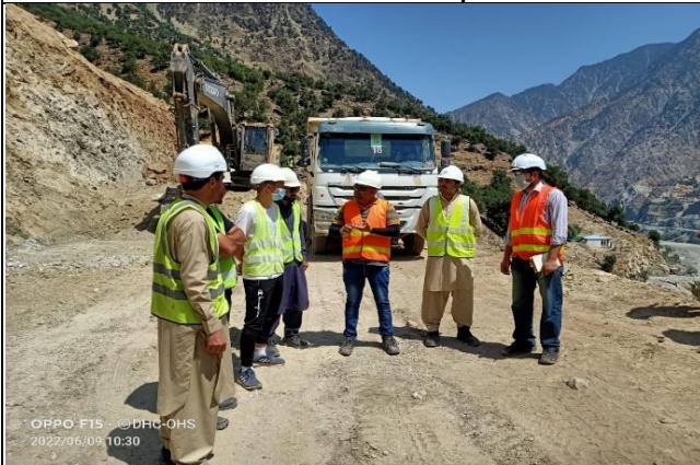
Weekly joint inspection of tripartite at RAR-01 bypass
