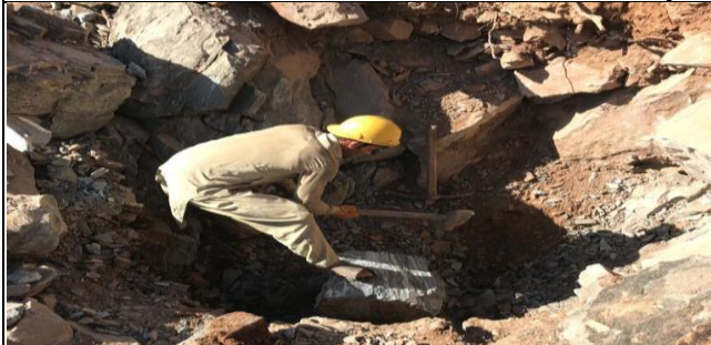
Excavation at T-111A
