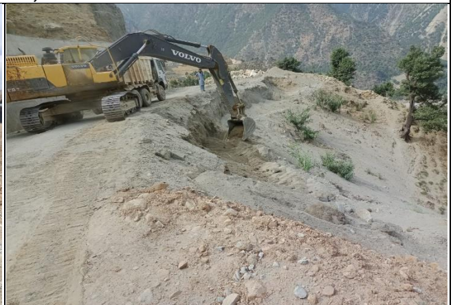
Excavation for Retaining wall foundation in Khushe at RD=K8+00
