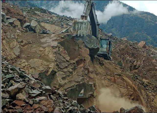
Excavation at K28 access Road KKH02
