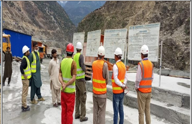
A view of joint site inspection with MCS consultant at CR2
