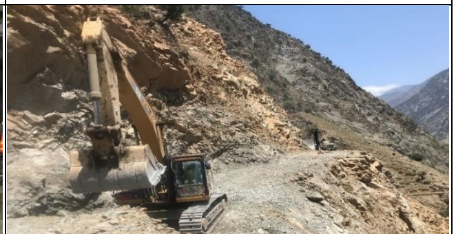
Excavation works at RAR-02
