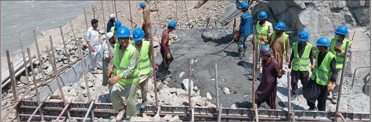
Concrete for foundation of Cableway Transportation System at K20+590 RAR02
