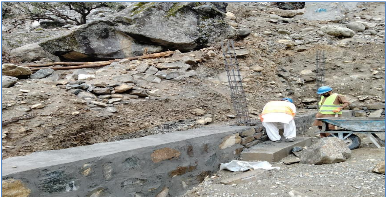
Terrace #2 boundary wall stone masonry was in progress
