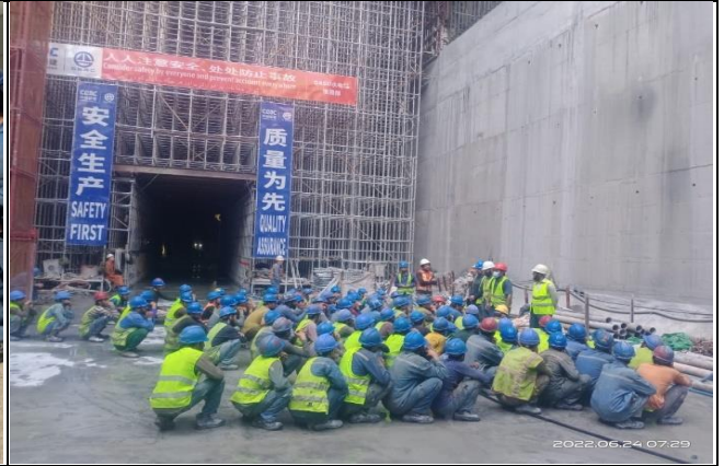
Daily TBT conducted by CGGC at DTB inlet
