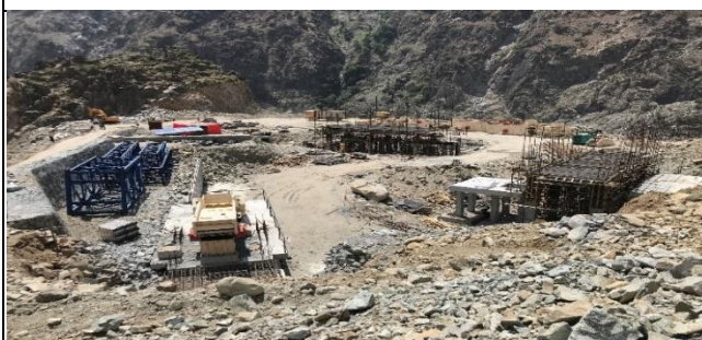
Civil Works at Uchar Crushing Plant
