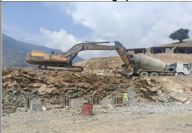
Concrete pouring for plant installation at K6+400 for Camp construction
