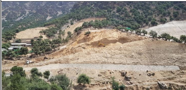
Excavation/Cutting work at Access road to Grid Station.
