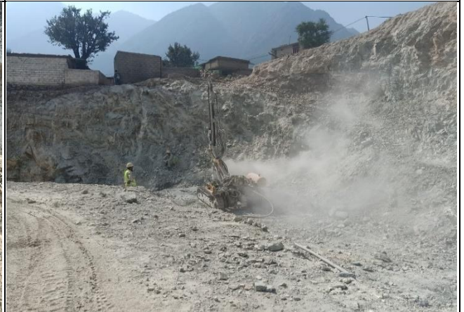
Drilling Work around K2+170 (Komila Bypass)
