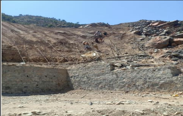
Slope Protection Of Nasirabad Site
