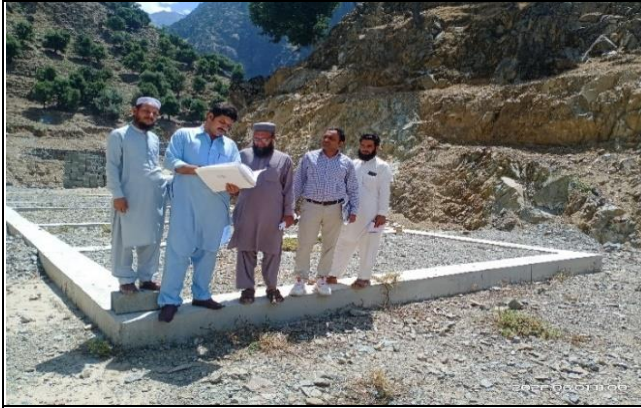
Field Verification visit of houses to Uchar Spoil dumping area on 1-06-2022
