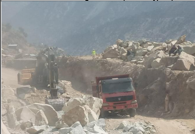
Excavation & Loading around K2(Komila Bypass)
