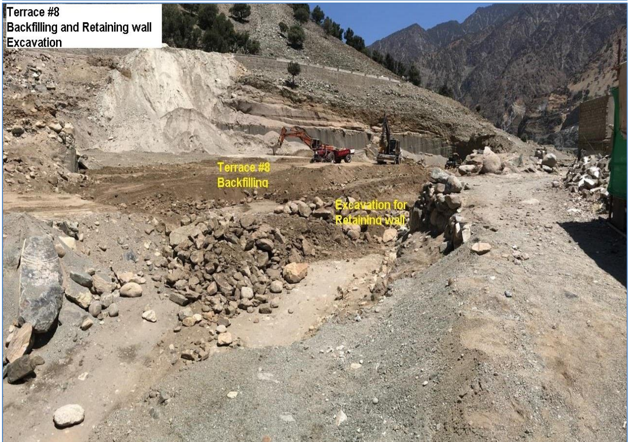
Terrace # 8 Backfilling / Compacting, Leveling and Excavation for Retaining wall
