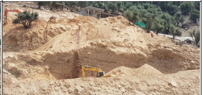
Excavation/Cutting work at Access road to Grid Station.
