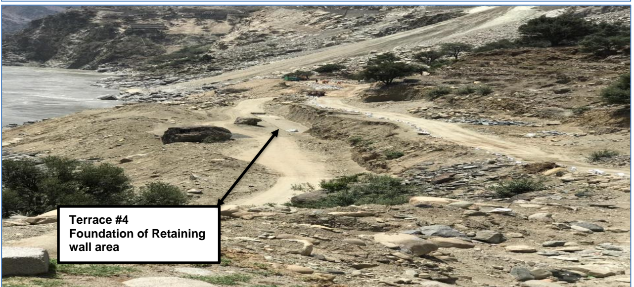
Terrace #4 Retaining wall area.
