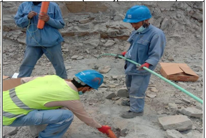
Charging for Blast at K13+254 RAR02
