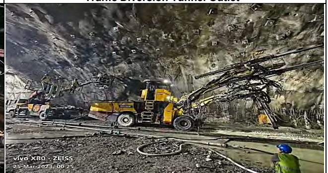
PH drilling and installation for PS tendon
