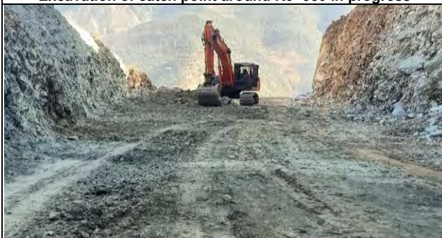
Sub grade Preparation in progress around K1+800
