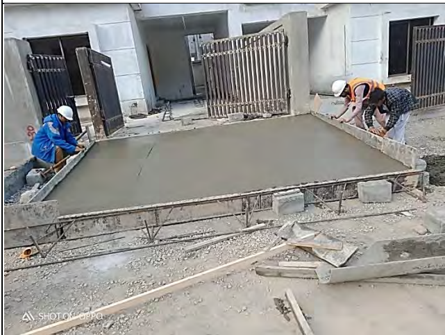
Cat 2 ramp concreting in progress
