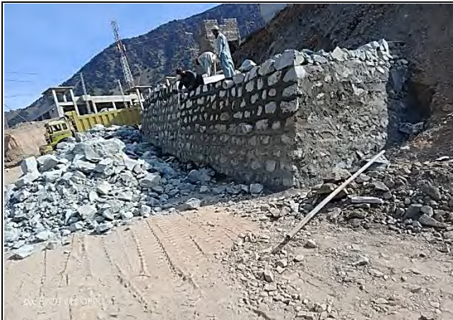
Stone masonry of breast wall along P1 road
