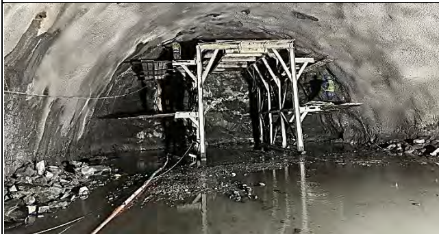
RT-02 US installation of wire mesh
