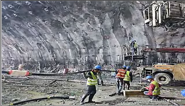
PH Installation of ps tendons
