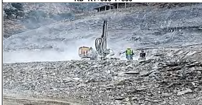
Excavation works at Zero Point 3rd bench
