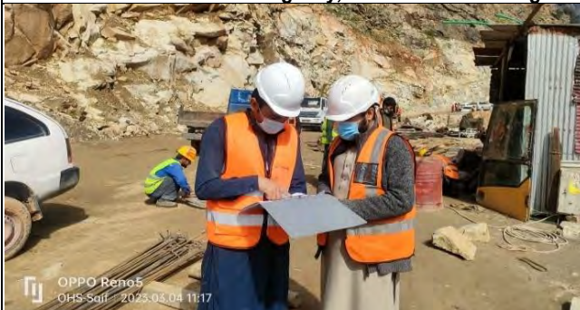
DHC OHS checking pre start hazard assessment at site
