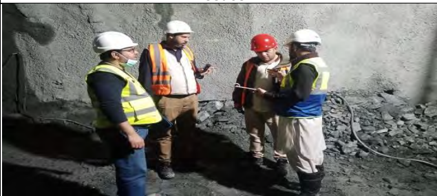
Tunneling GAP Analysis conducted by DHC OHS and CCECC OHS
