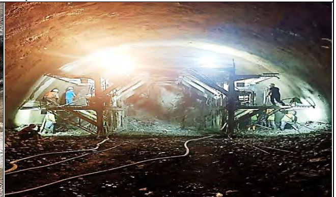
Drilling for blast Logro-A RD=K9+426-9+430
