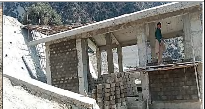
Block masonry at mosque is in progress
