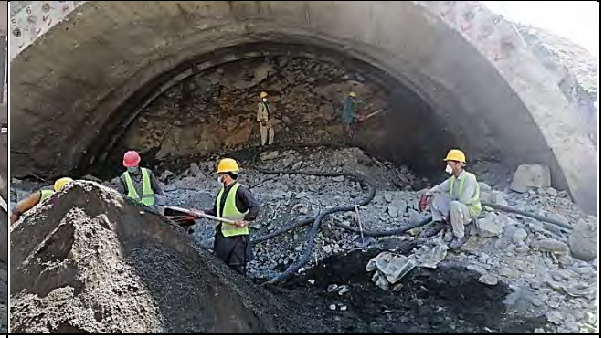
Dugah tunnel K23+647 2nd layer shotcrete
