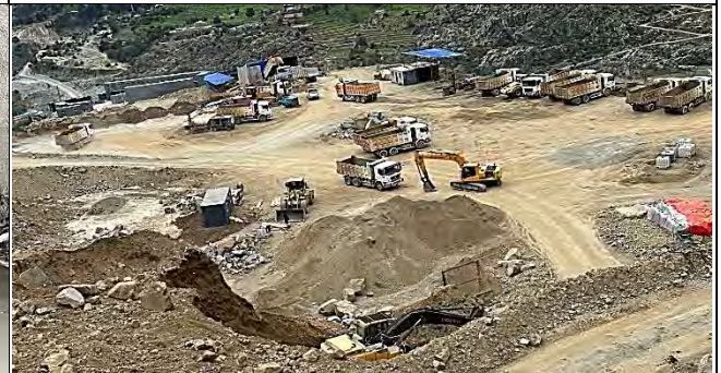
Switchyard excavation & mucking
