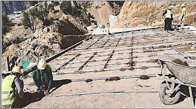
Roof treatment of Control House building
