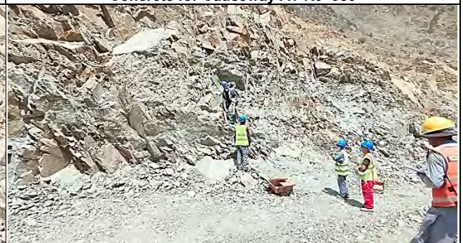
Charging for Blast at K12+990 ~ K13+050
