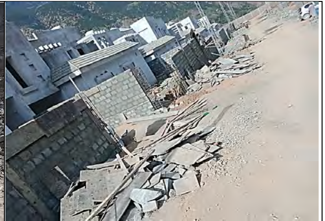
Block masonry for the boundary wall at Cat 2C
