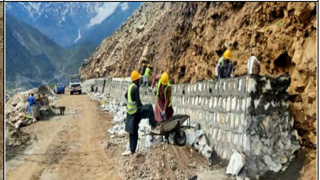
Stone Masonry B/Wall in progress around K0+800
