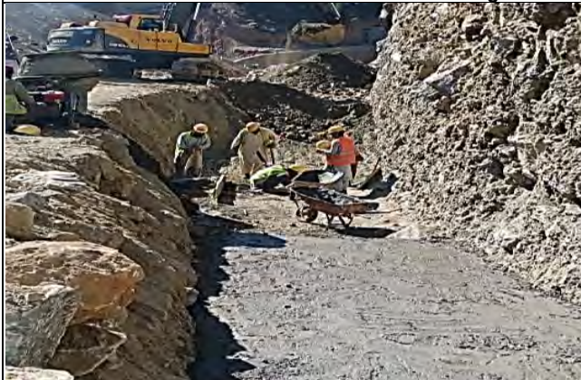
Base concrete of Breast Wall at access road
