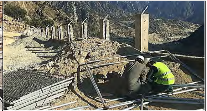
Frame cutting and fixing on Fence Wall
