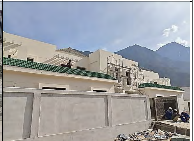
Painting at cat 2A in progress
