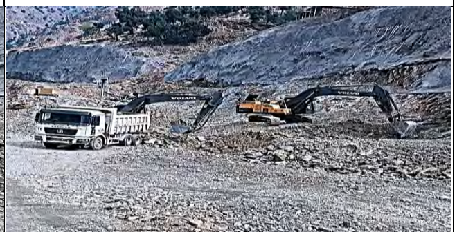
Excavation works at Zero Point 3rd bench
