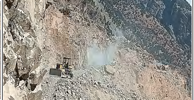
Excavation at K34 Access Road
