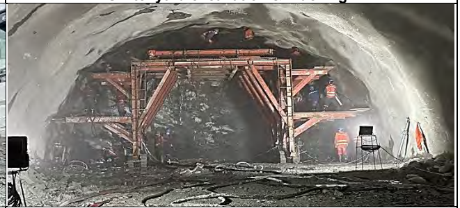
TRT-01 US Drilling for blast
