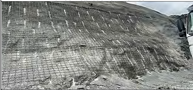
Switchyard Installation of wire mesh
