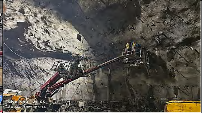
PH PS tendon installation
