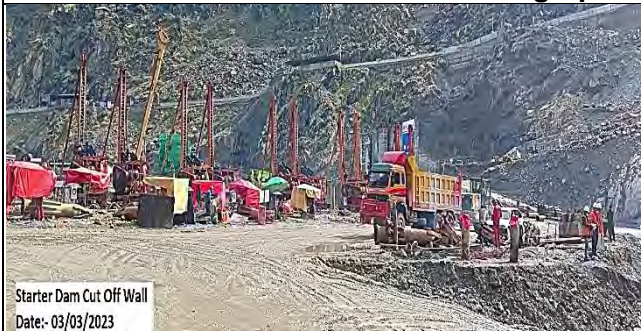
Starter Dam Cut off Wall
