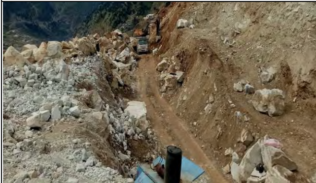
Excavation of catch point around K0+550 in progress
