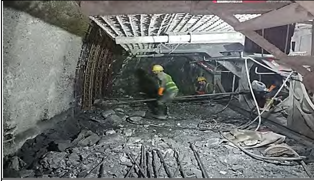
Drilling for rock bolts at K4
