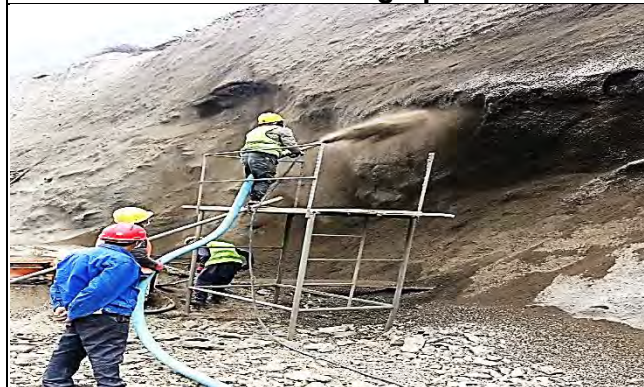
Shotcrete for slope protection at Zero Point 3rd Bench RD=K1+800-1+850
