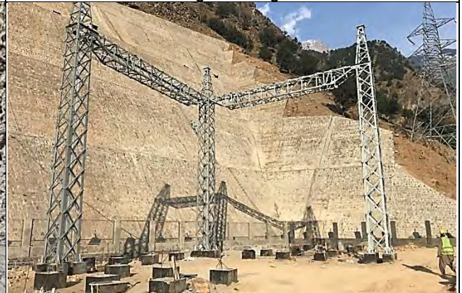
Erection of Gantry on terrace-1 of Grid Station
