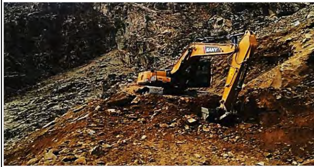
Excavation at K28 access Road
