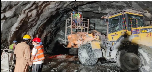
TRT-01 (U S). Grouting for rock dowels
