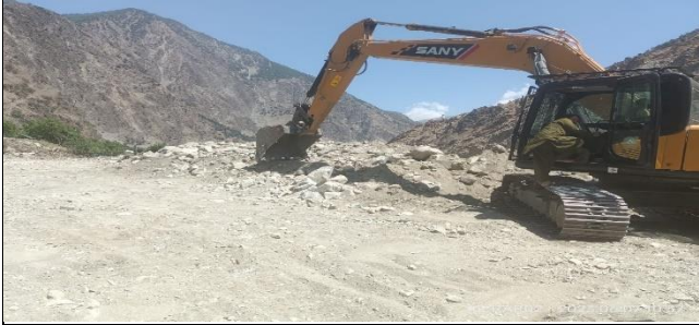
excavation at K34+600
