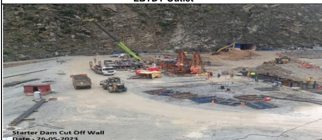
Starter Dam Cut Off Wall
