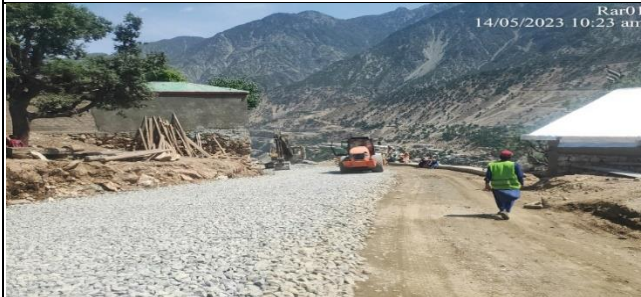
Laying & Compaction of water bound macadam (Komila)
