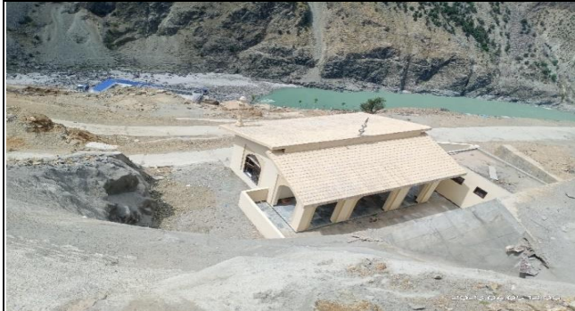
New constructed mosque at Rv nasirabad-01
