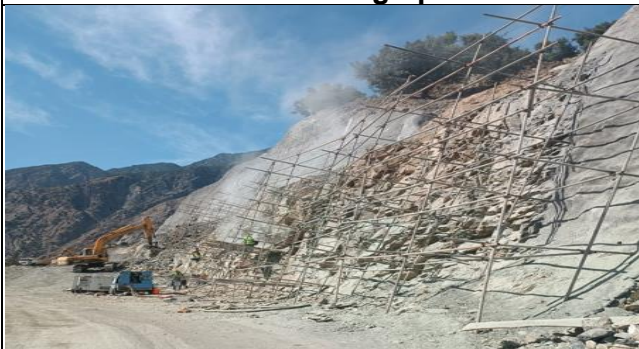
Slope Protection works at K1+700
