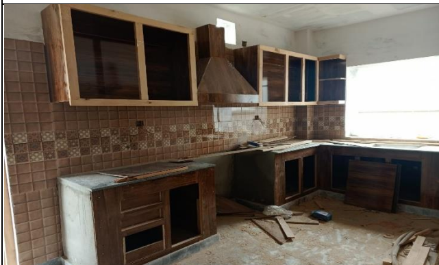
Kitchen cabinet work at cat 2 is in progress
