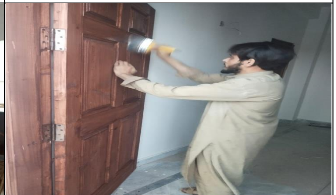
Door poishing work cat 2
