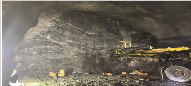
Access below surge chamber (A 1st Round) Charging for blast
