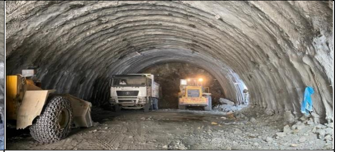
Tunnel Support Works K23+598
