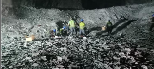
LPT-1 charging for invert blast
