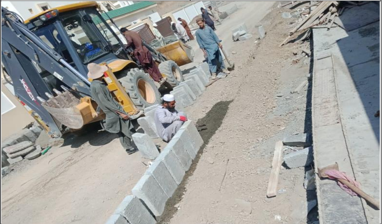
Fixing of curb stone along s1 road
