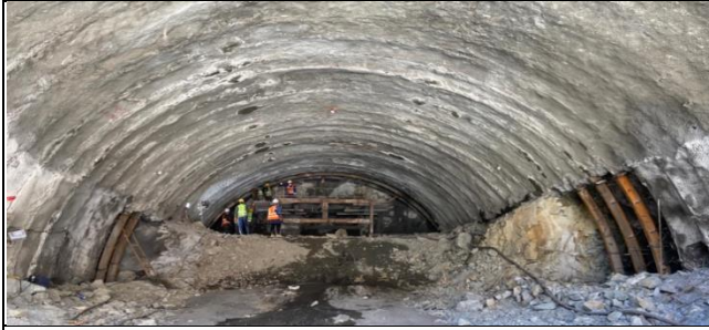
Tunnel Support Works K11+831
