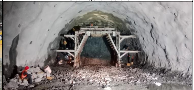
TRT01 charging for blast
