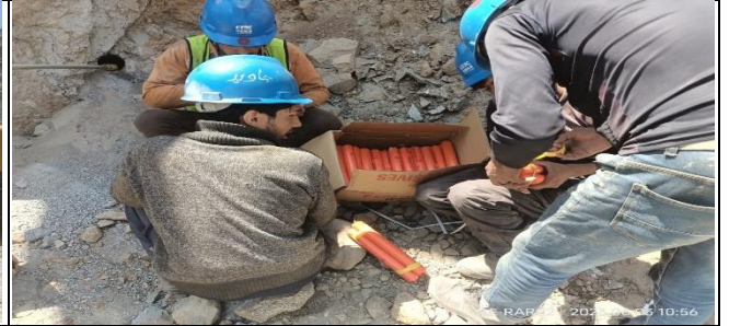
Charging for Blast at K12+990 ~ K13+050
