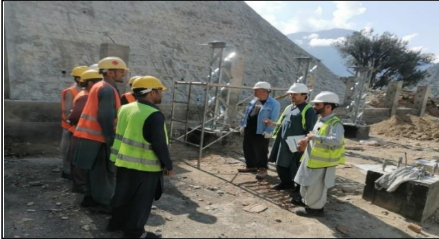
Discussion on safety implementation and improvement at Grid Station site.
