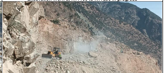
Excavation at K40 Access Road
