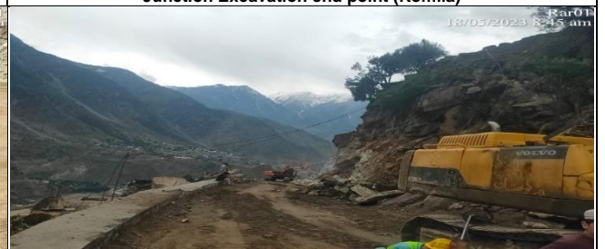
Excavation Work at K1+100 to K1+250 in progress
