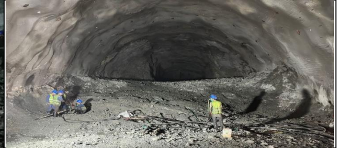
PAT-01 Invert drilling for blast
