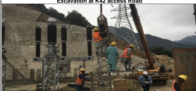
Installation of switch gear equipment on Upper terrace of Grid Station
