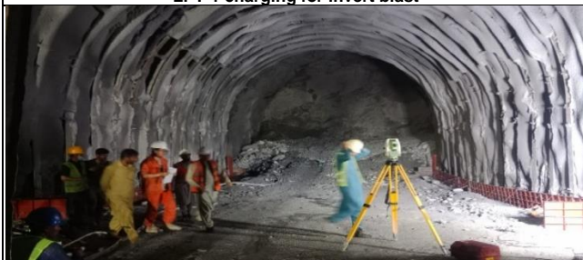
PAT02 Survey for formwork.
