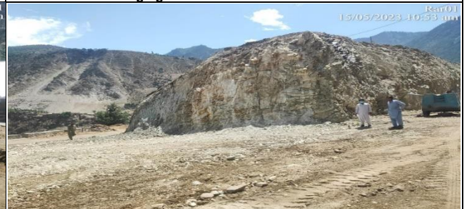
Junction Excavation end point (Komila)
