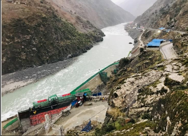
MW01_Inlet of Diversion Tunnels A & B
