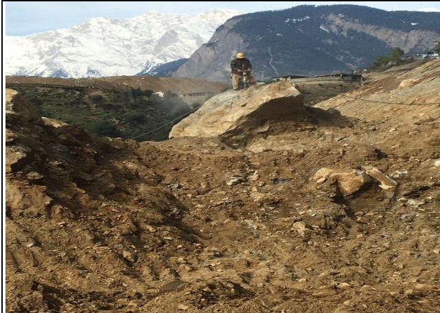
Drilling work on access road to Grid Station
