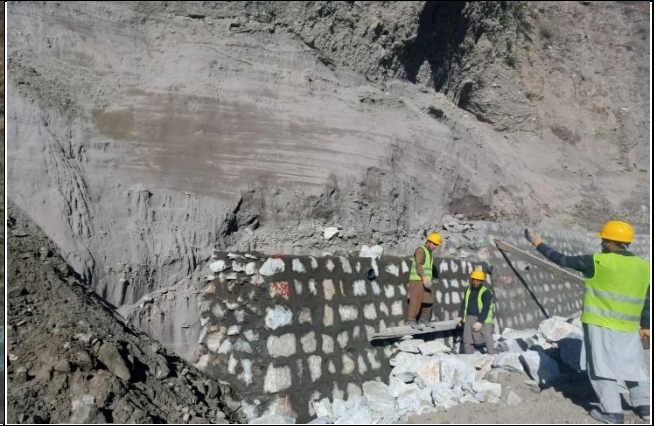
Breast Wall at K0+130 in progress (Komila Bypass)
