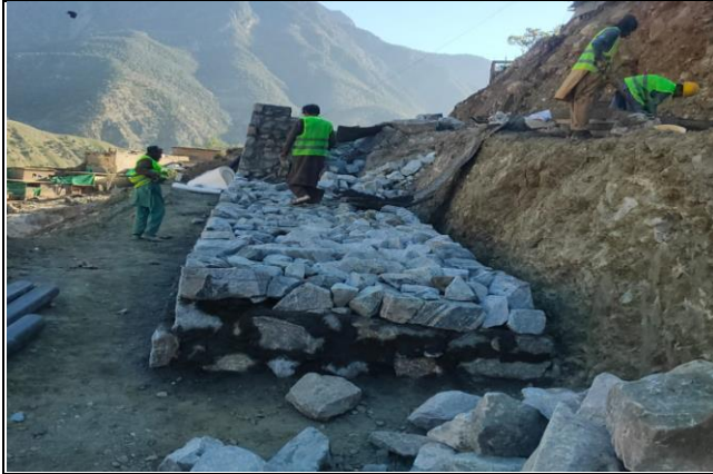
Retaining Wall in progress K1+800 (Komila Bypass)
