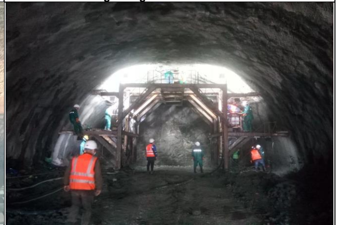
Drilling for Blast in Logro-A Tunnel RD=K9+206
