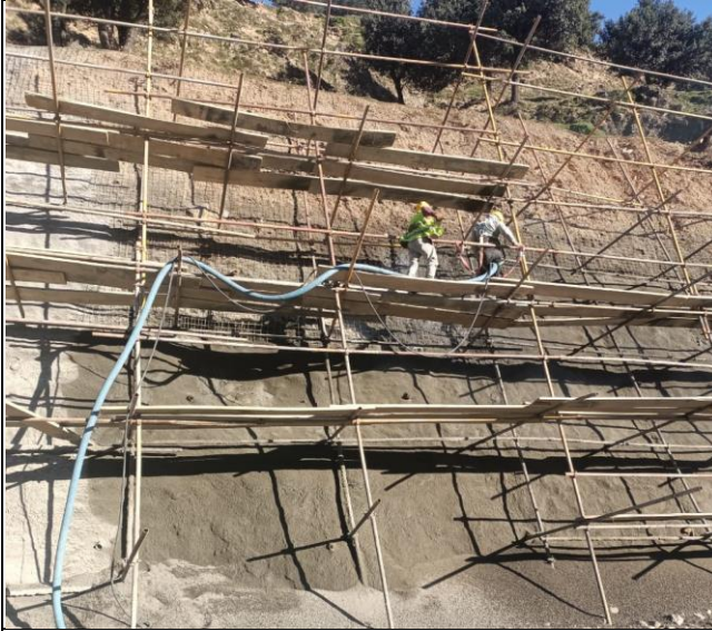
Shotcrete at Zero Point Third Bench RD=1+450
