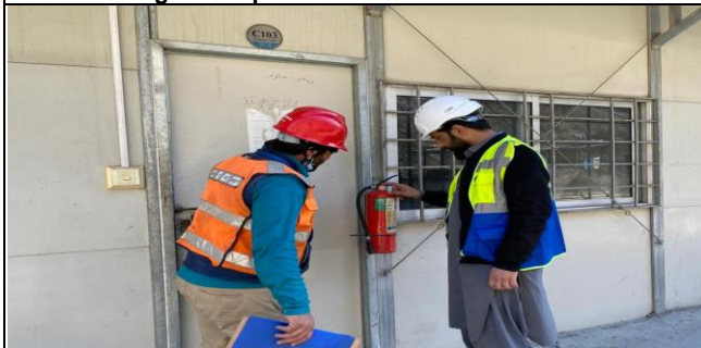
During AFI inspection of portable fire extinguisher at MW02
