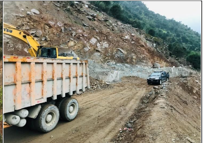
MW-02_Excavation at Intake Area 990m
