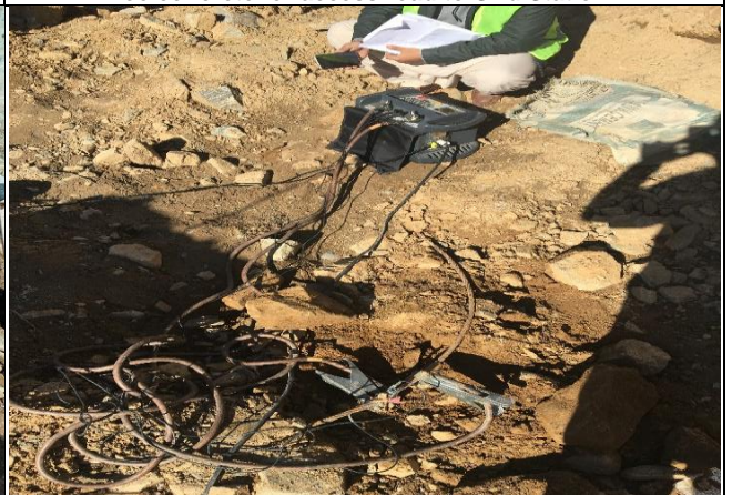
Connectivity test of copper wire with exothermic welding in Grid Station.
