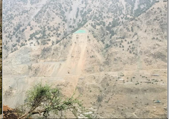
MW01_Excavation for Right Bank Cable Crane
