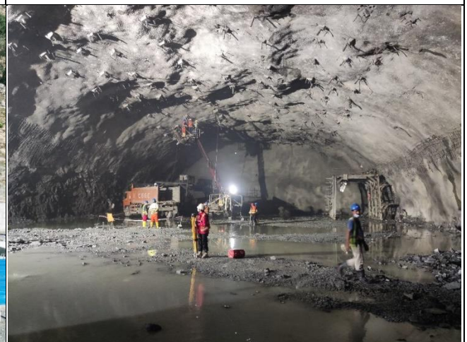
MW-02-Excation Additional Support Work in Powerhouse Cavern
