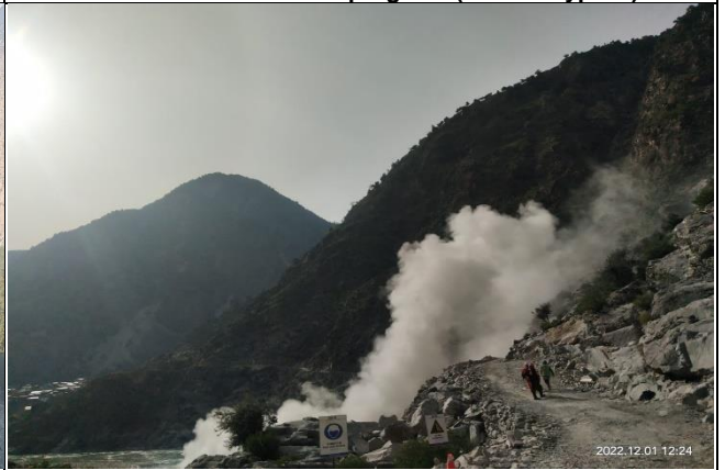
Blasting at Seer Gayal Access Road
