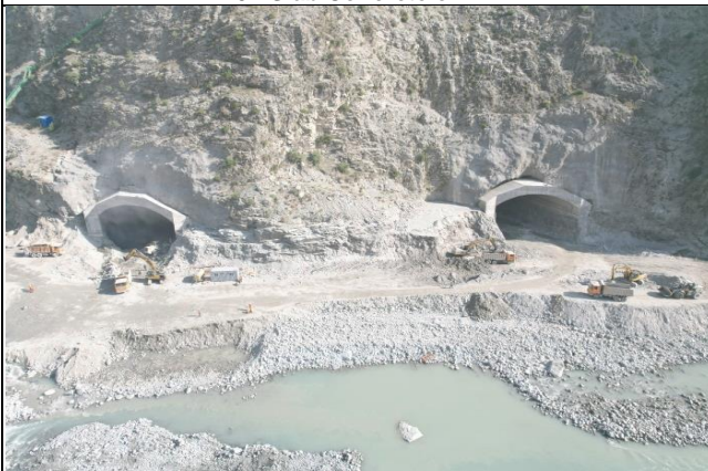
MW01-Diversion Tunnel A&B – Outlet Structure
