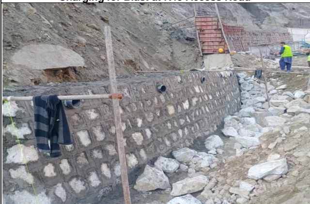
Breast Wall in progress start section (KOMILA BYPASS)
