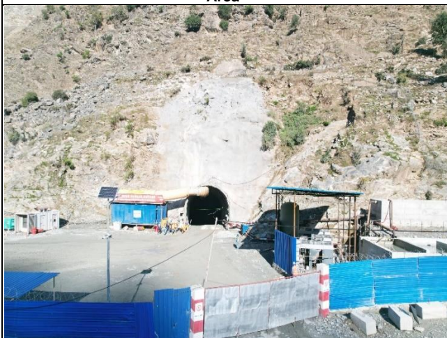
MW-02-Adit Tunnel CT-2 for Excavation of Tailrace Tunnels
