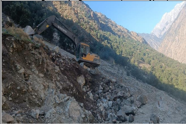
Excavation at K33+800 RAR02
