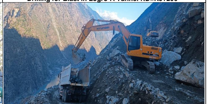
Excavation and Hauling at K31+100 KKH02
