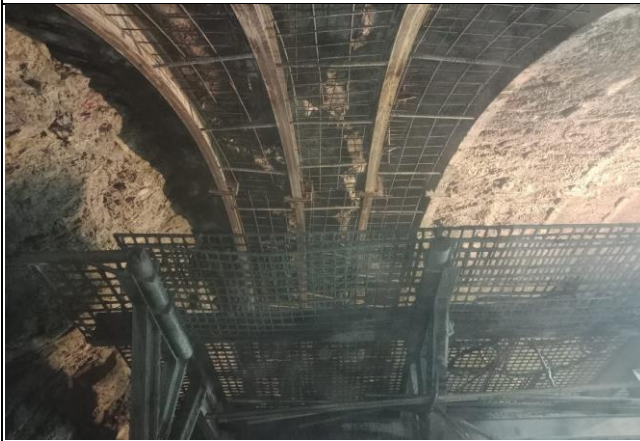
Primary Support works in K4 tunnel in progress
