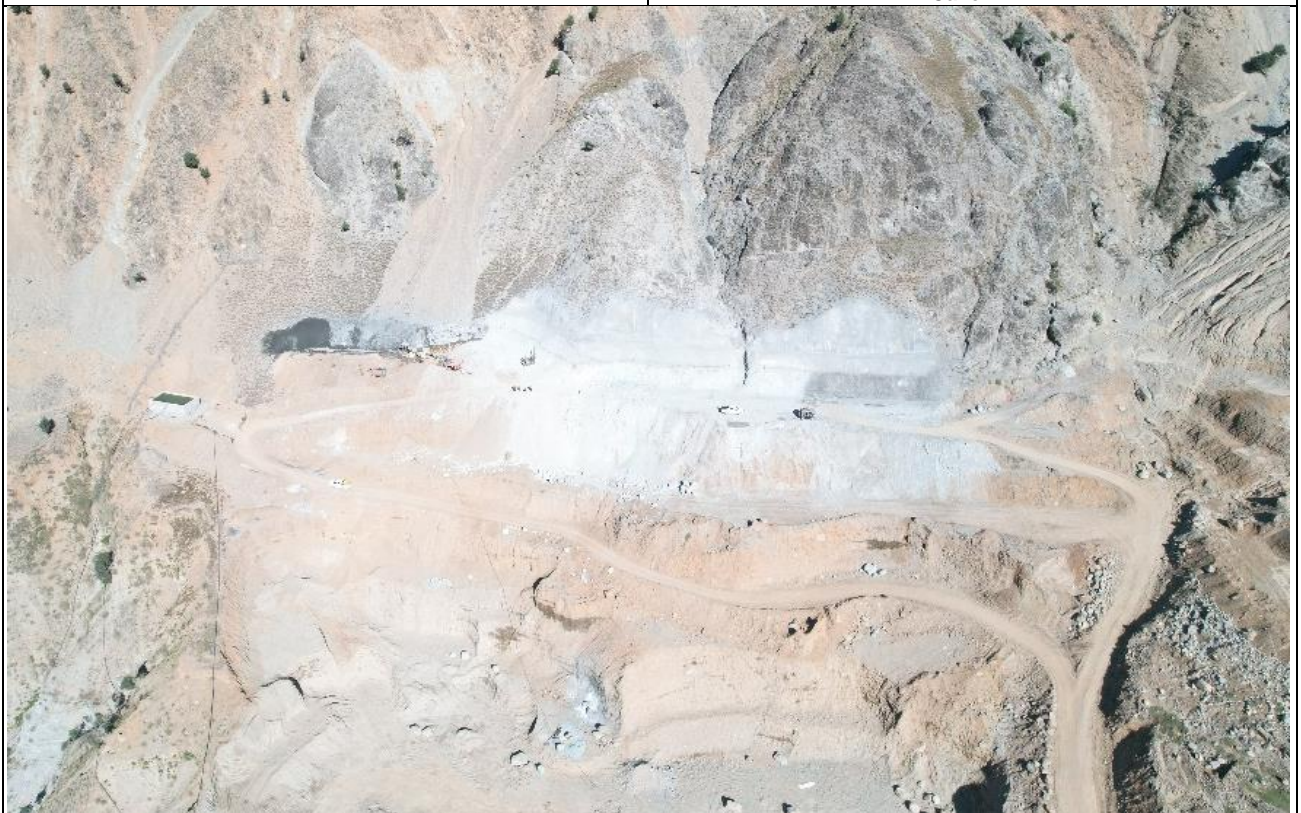
MW-02-Excavation and Slope Protection works at Switchyard of MW-02
