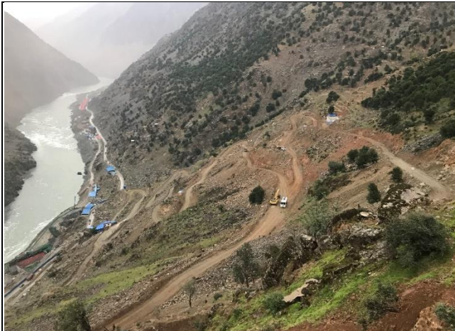
MW02_Access Road for Left Bank Cable Crane and Intake Area
