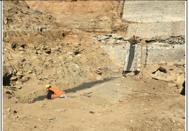
Toe concrete for access road to Grid Station
