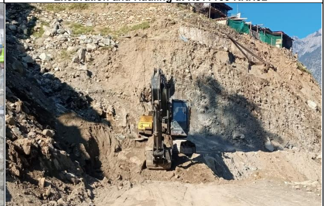
Excavation work in progress at K0+350 (KOMILA BYPASS)
