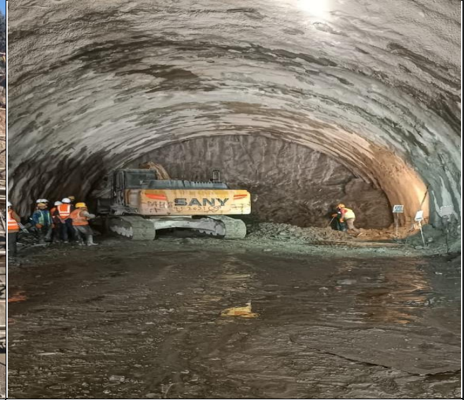
Mucking in Logro-A tunnel RD=K9+206
