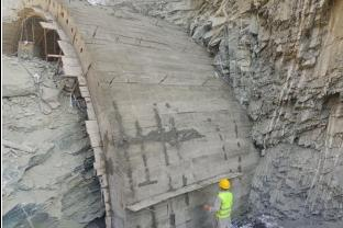
Serial arches concrete works at K4 tunnel outlet Portal
