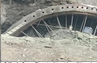
Drilling for Conopy Pipes at outlet portal area K4 tunnel
