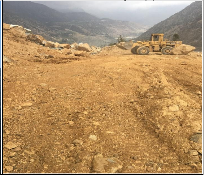
Excavation/Cutting work at Access road to Grid Station.
