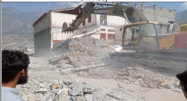
Demolishing of Local houses (Komila Bypass)
