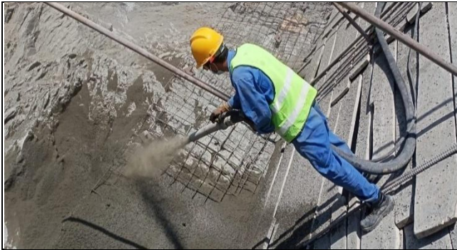
Shotcrete for 2nd layer at K4 tunnel outlet area.
