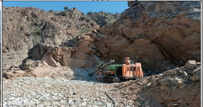
Drilling at K28+620 KKH02
