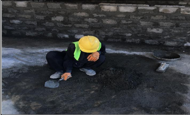
Block masonry work in Control House building
