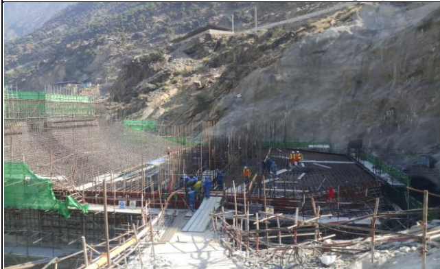
MW-01: Inlet of Diversion Tunnel-B
