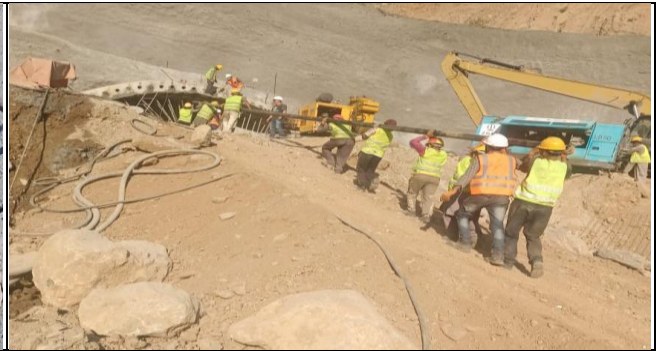
Installation of Canopy pipes at logro-A inlet.
