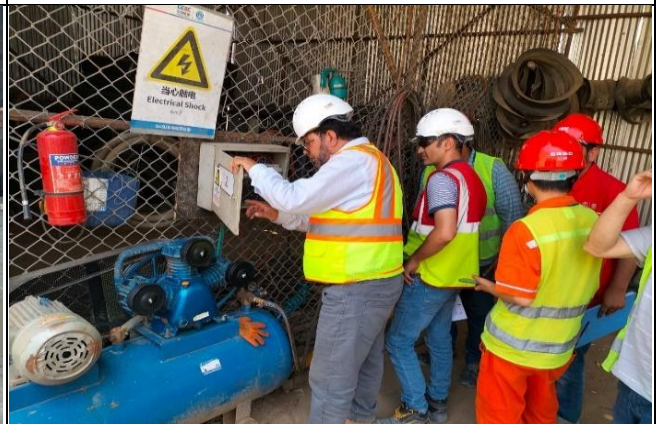
Elcetrical Inspection carried out by DHC OHS at CR9
