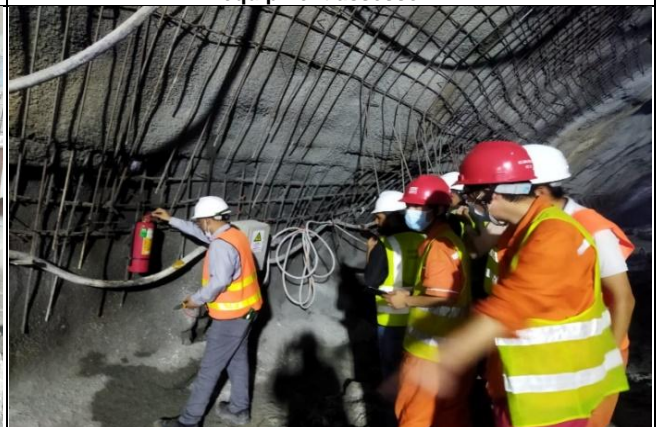
Fire extinguisher inspection conducted during joint inspection visit
