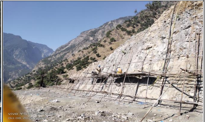
MW-01: Excavation for Right Bank Cable
