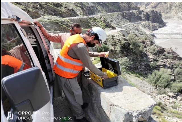
First aid box inspection conducted by DHC OHS at KKH-02 works
