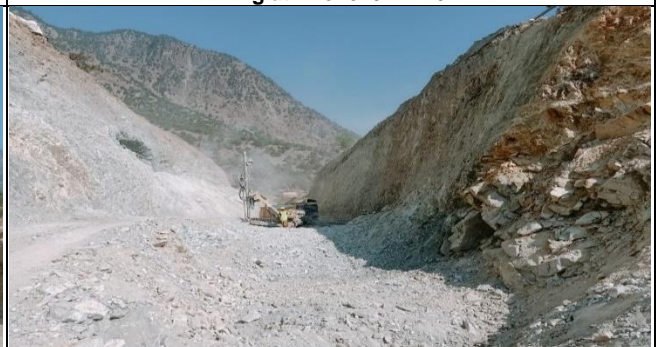
Drilling for Blasting K2+160 (KOMILA BYPASS)
