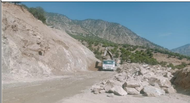
EXCAVATION & LOADING K2+120 in progress (KOMILA BYPASS)
