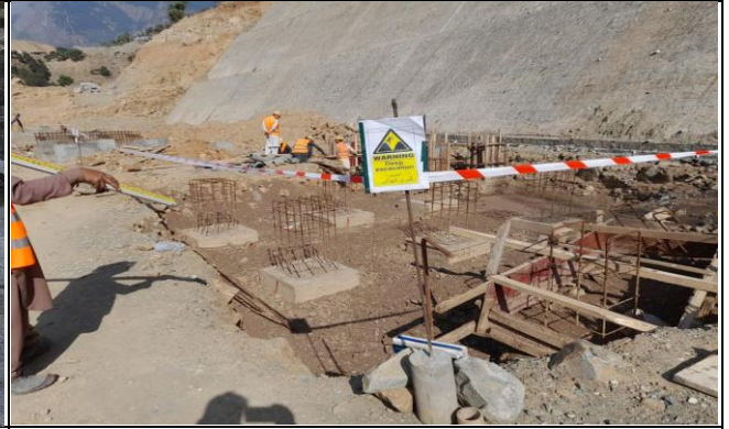
Foundation concrete of switch gear equipments
