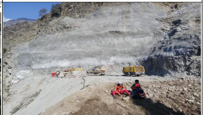
MW-01: Excavation at Outlet of Left Bank Traffic Diversion Tunnel.
