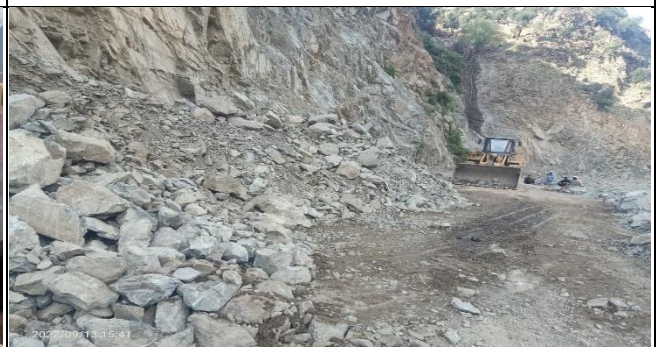
Removing of Slided Material around K11+700 (RAR-01)
