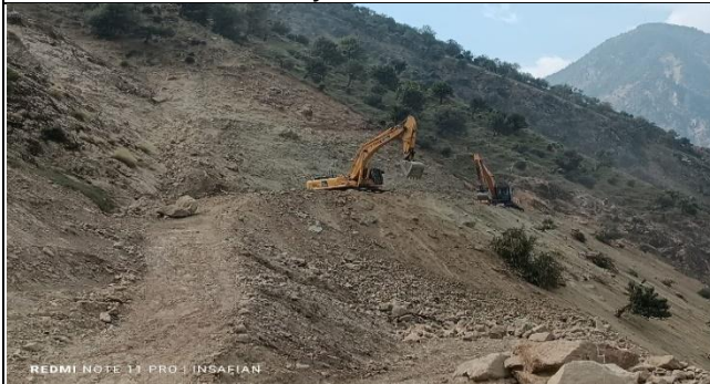
Excavation at K31+200 KKH02
