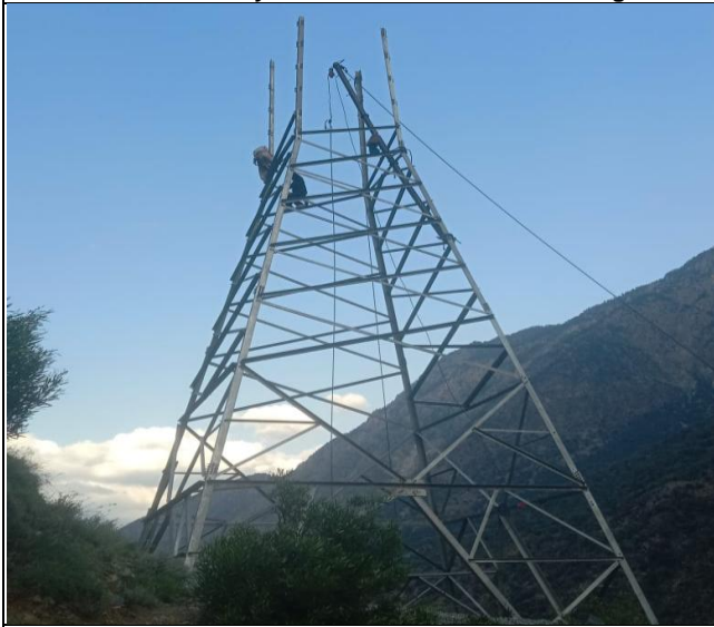
Tower erection at T-139A
