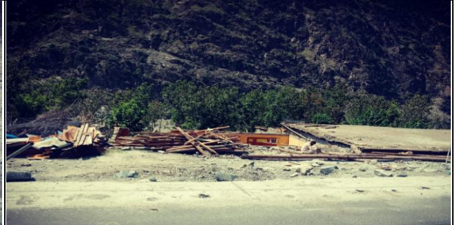
A picture of dismantled house in Barseen village
