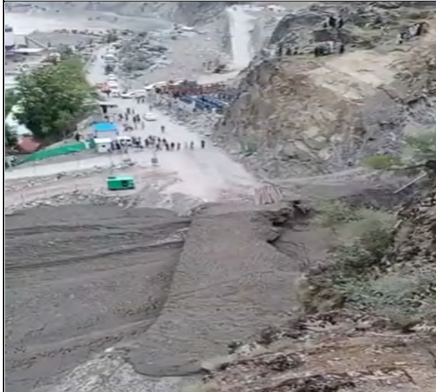
Debris flow at overtopples uchaar nullah bridge
