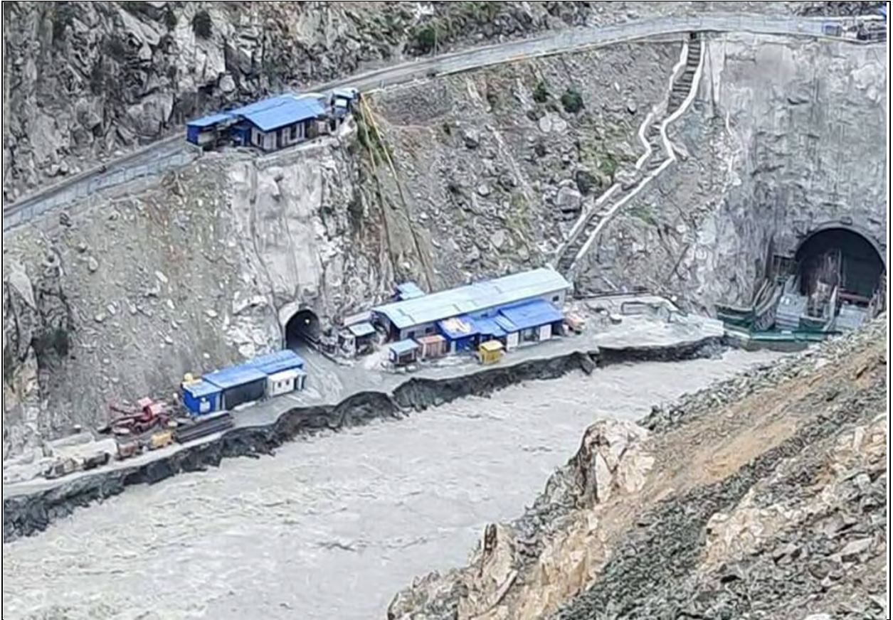
Scoured CR-02 area-Flood of 27 th July 2022
