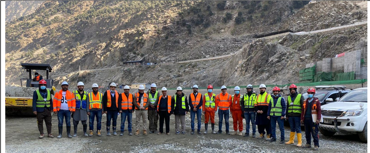
WB Visit to DHPP K-09 Tunnel and Cofferdam Site on 22 nd of Dec 2022
